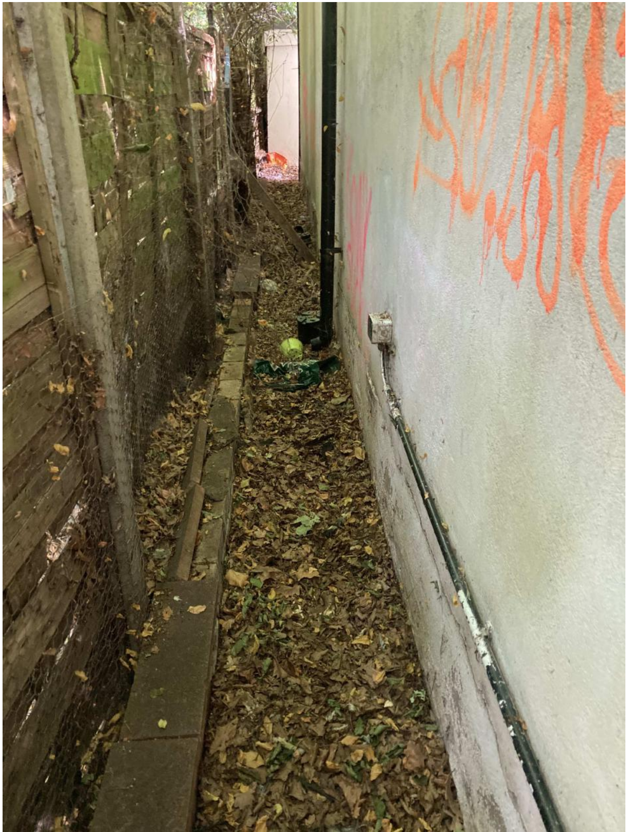
The rear boundary with Coldfall is demarcated by a low brick wall and fence.
