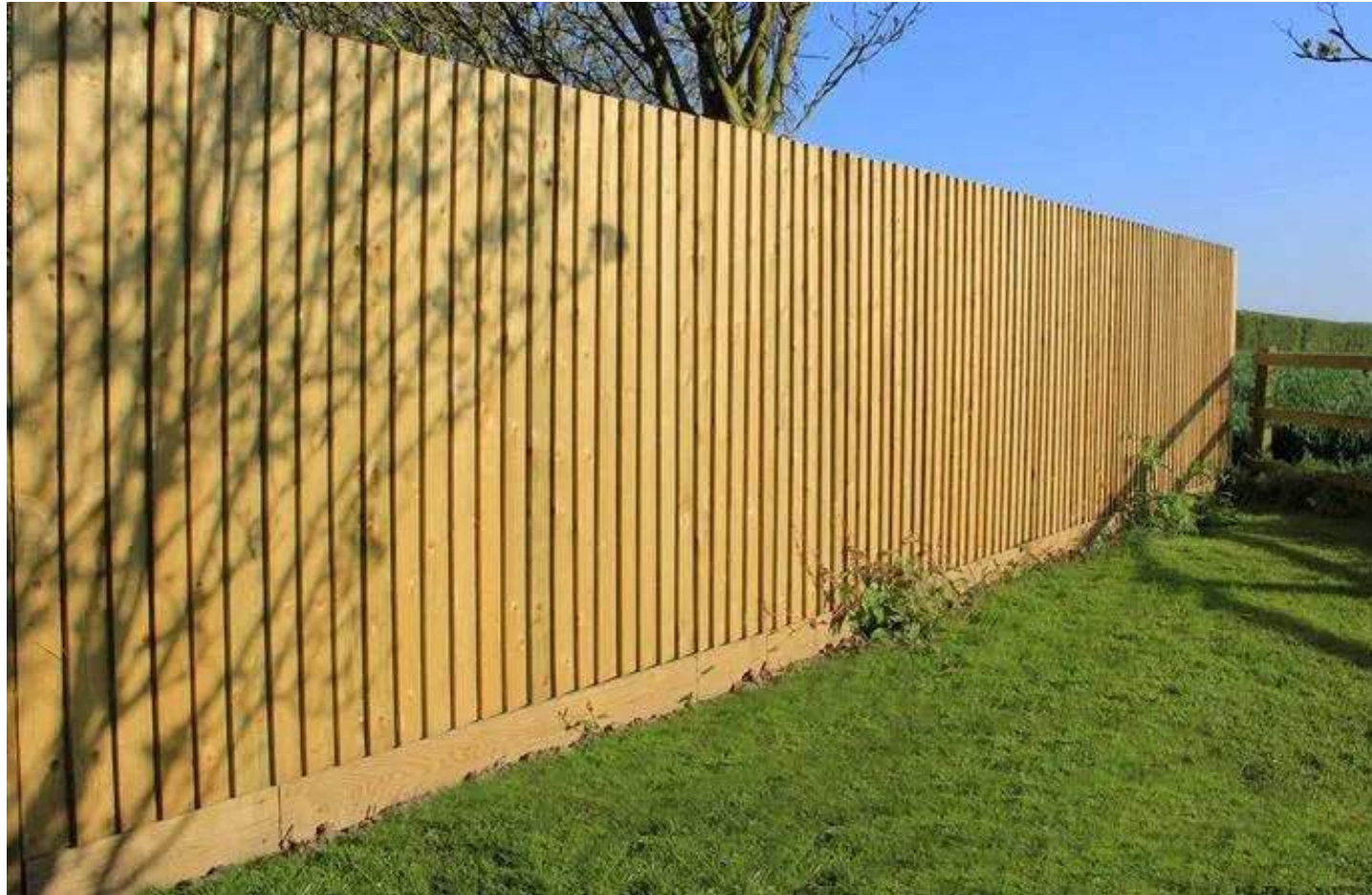
Traditional featherboard fencing
