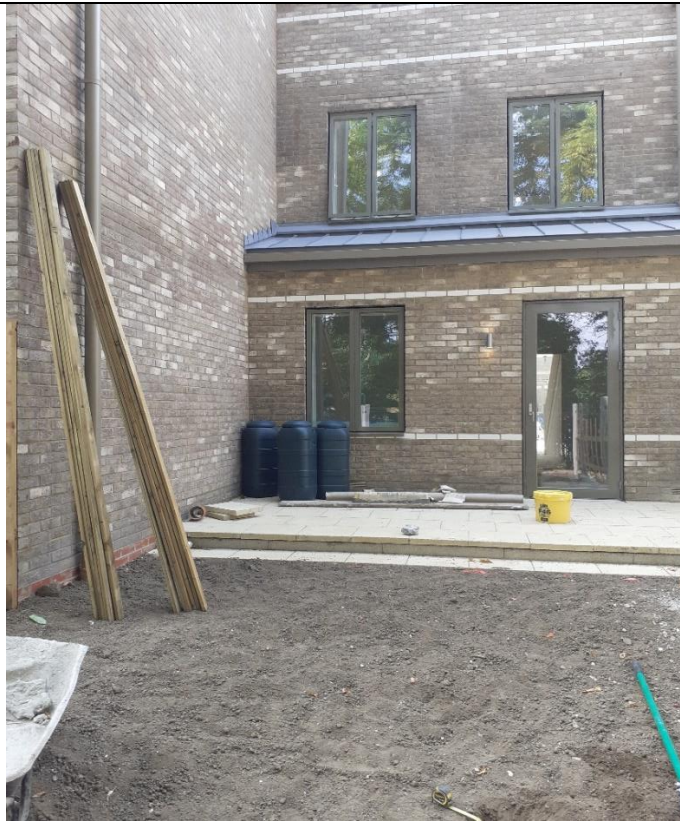
Plate 11: Plot 52 (Block A) general view.
