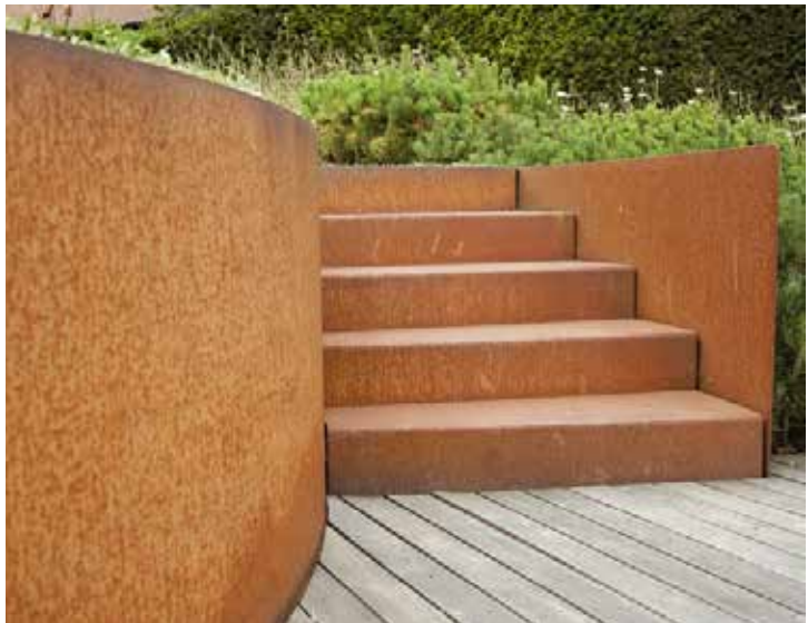
Corten steel walls
