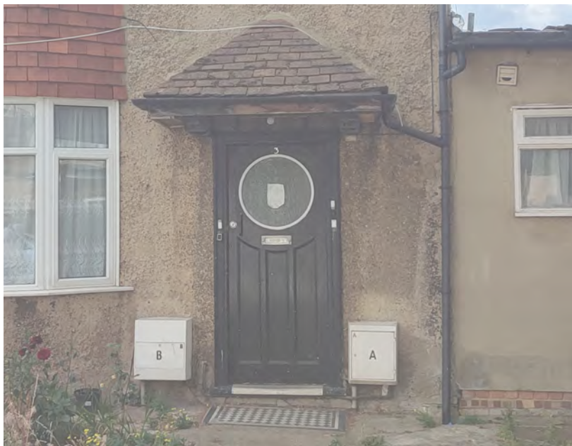
Front communal entrance door
