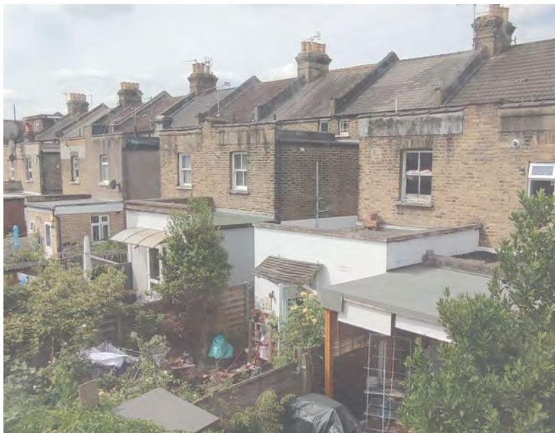
West neighbouring properties from first floor rear diagonal window
