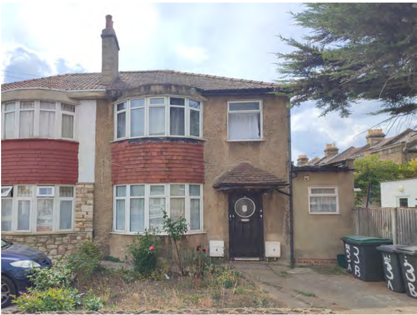
Front Elevation Photograph showing material pallet
