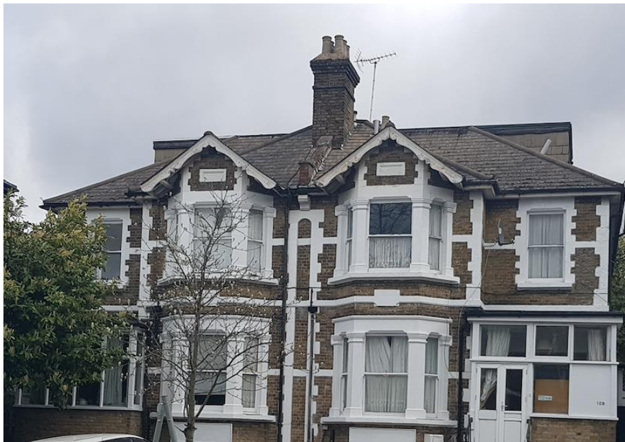
Front of 108-110 Colney Hatch Lane – showing existing front extensions to each property.
