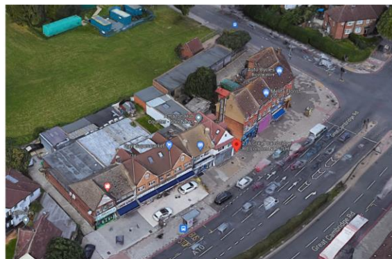
6. Front Aerial View of Site at Cambridge Road
