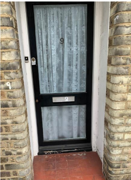
Figure 5: No.9 Front Entrance Door
