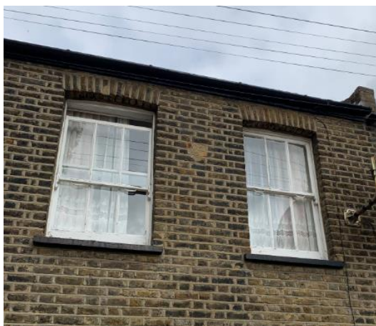
Figure 1: No.6 First Floor Front Elevation Windows
