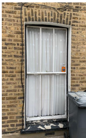
Figure 2: No.9 Ground Floor Front Elevation Window
