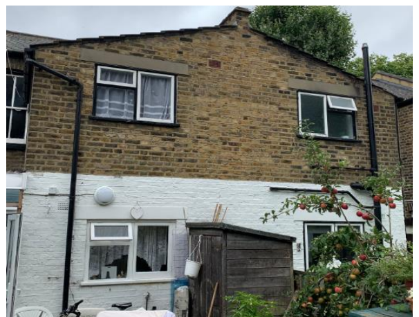
Figure 3: No.7 & 8 Rear Elevation Casement Units
