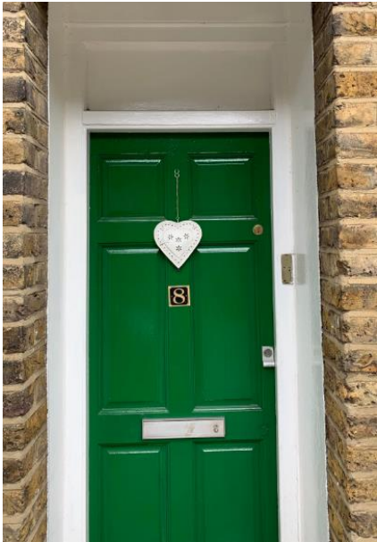
Figure 4: No.8 Front Entrance Door
