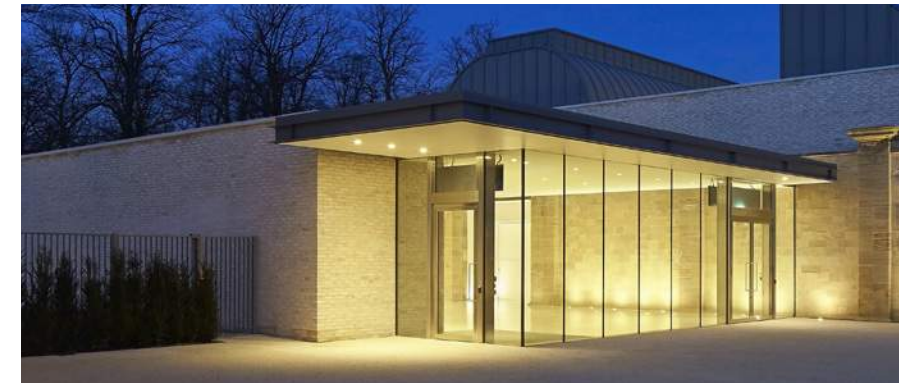
Figure 8.23: Architecture - Lighting to specific architectural details such as soffits and canopies.
