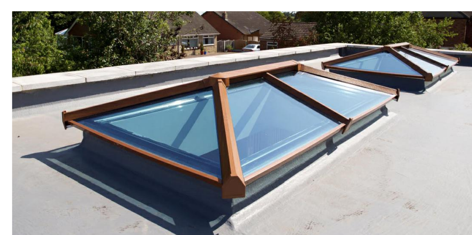
LANTERN LIGHT TO OUTBUILDING FLAT ROOF.
