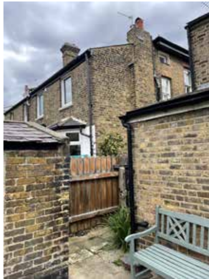
South-east corner of No. 6
