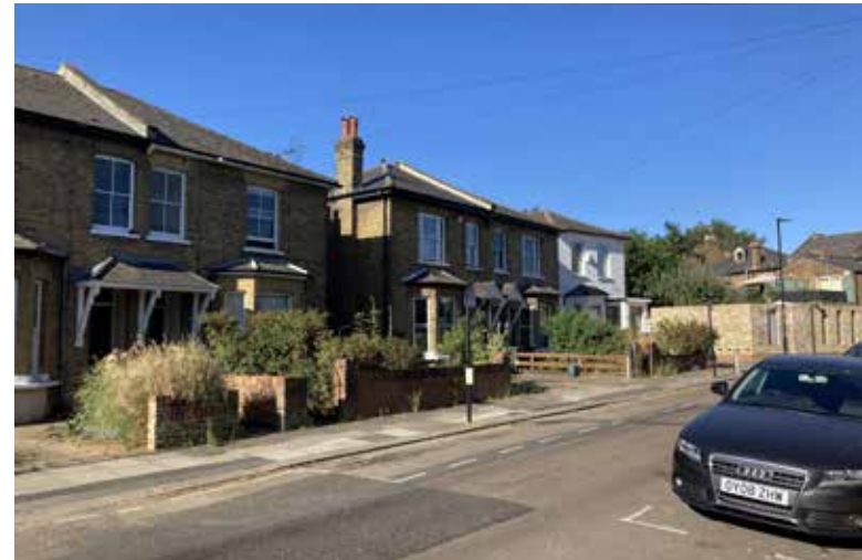
No.s 2 to 8 Thorold Road, works to new-build house at 44 Whittington Rd underway
