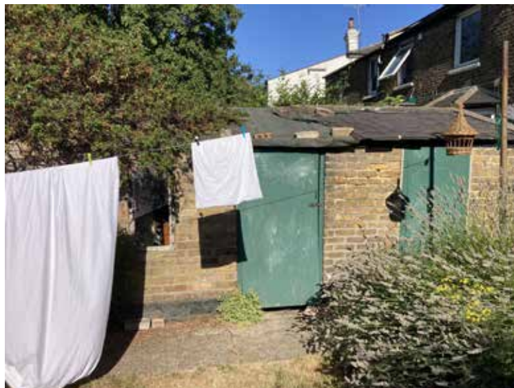
Out building close to main house
