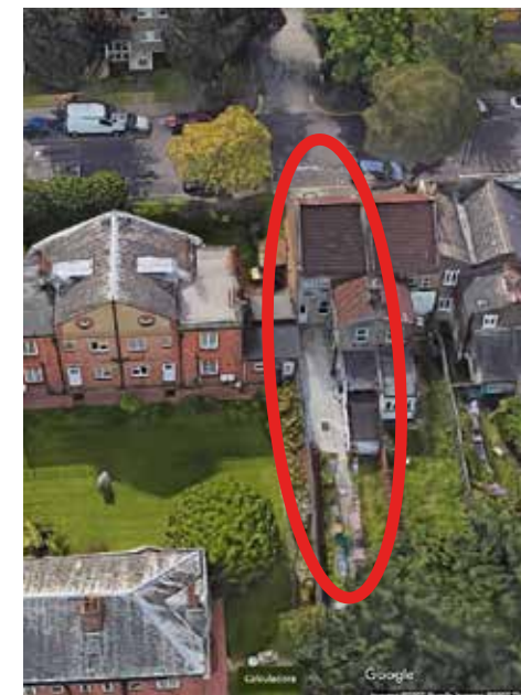
Existing aerial view of 26 Nightingale Rd
