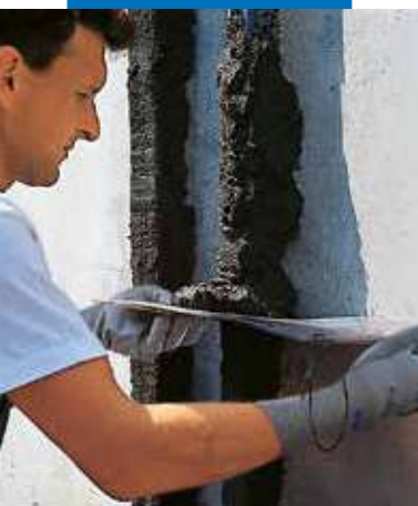
Creating the required form with a template
