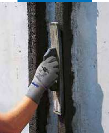
Finishing with a sponge float
