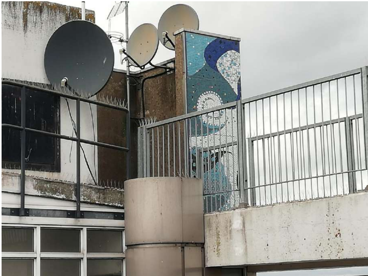
In-situ-reinforced concrete panel supporting mosaic at roof level
