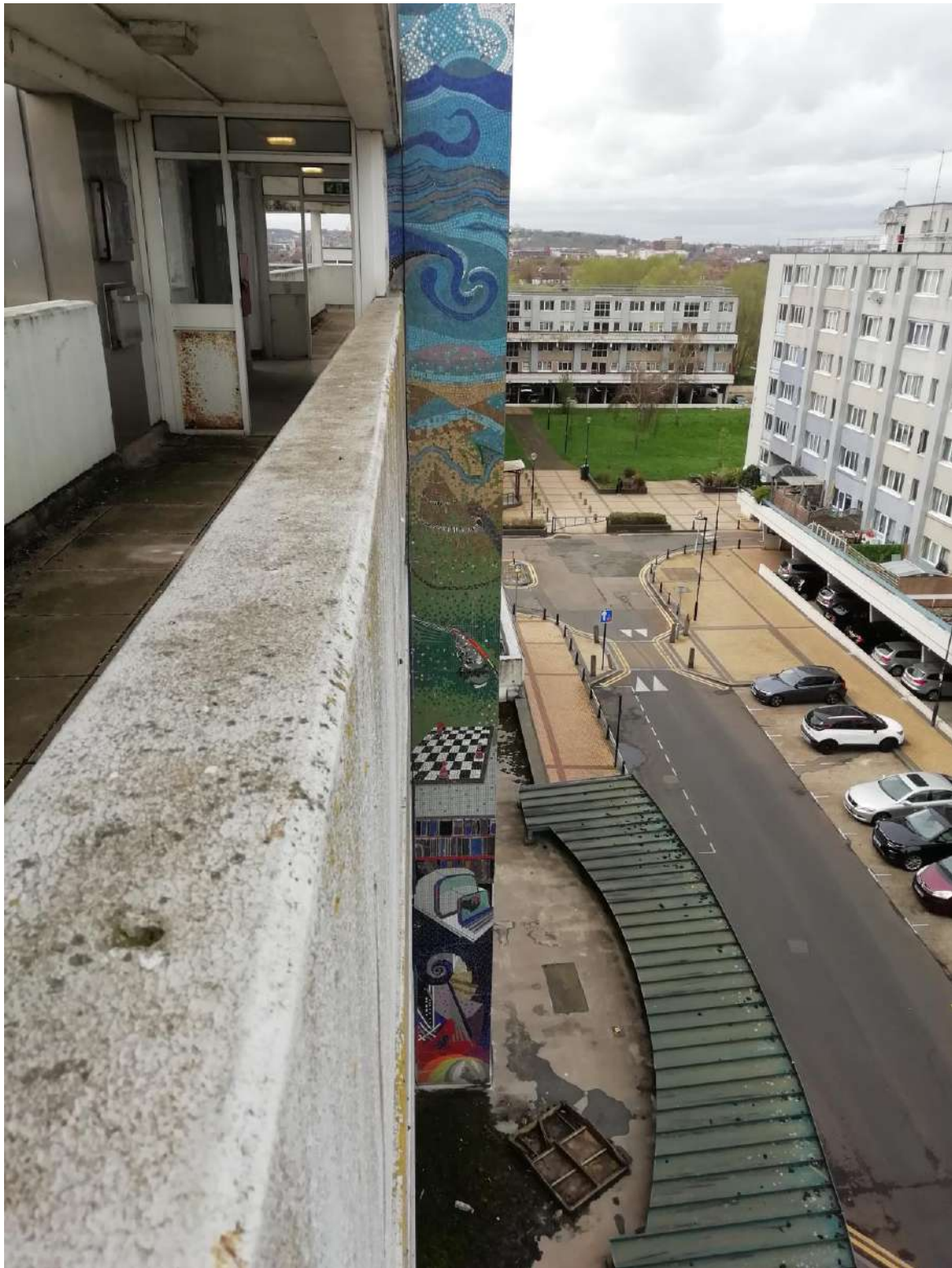
6 th Floor Level – Viewed from Walkway
