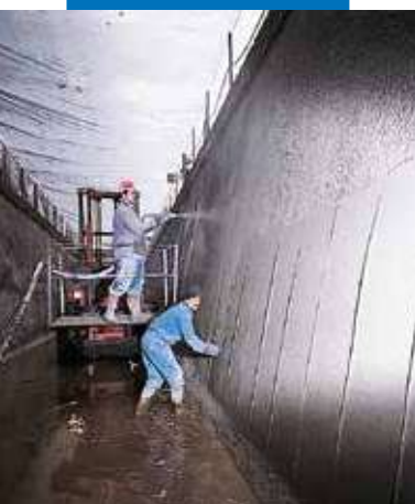
Bertini hydroelectric canal - Robbiate (Como) - Italy: finishing with a trowel
