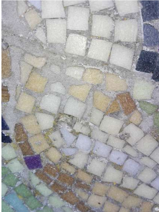
Images 3a-b – “Opaque”effect due to hight presence of limescale plus whitening of cement carbonation
