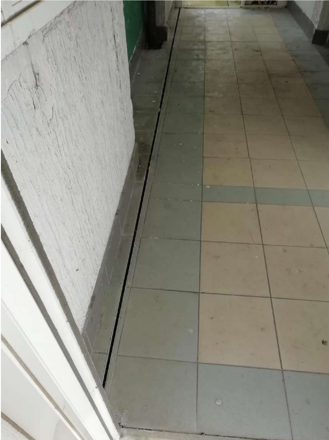
Landing Slab/Walkway Junction
