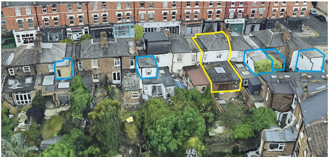
Rear 3D view of terrace along Park Road (ref. Google Earth)
