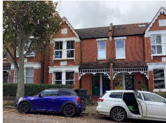
Front elevation of main property
