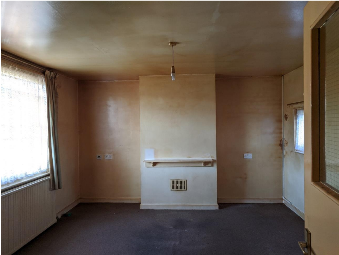
Photograph 5 - Internal condition of 1st floor Almshouse with boarded fire place (No 19)
