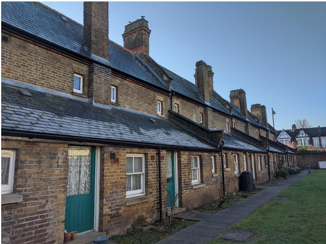
Photograph 2 - Rear view of existing Almshouses
