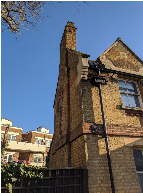
Photograph 4 - Gable wall to Almshouse
