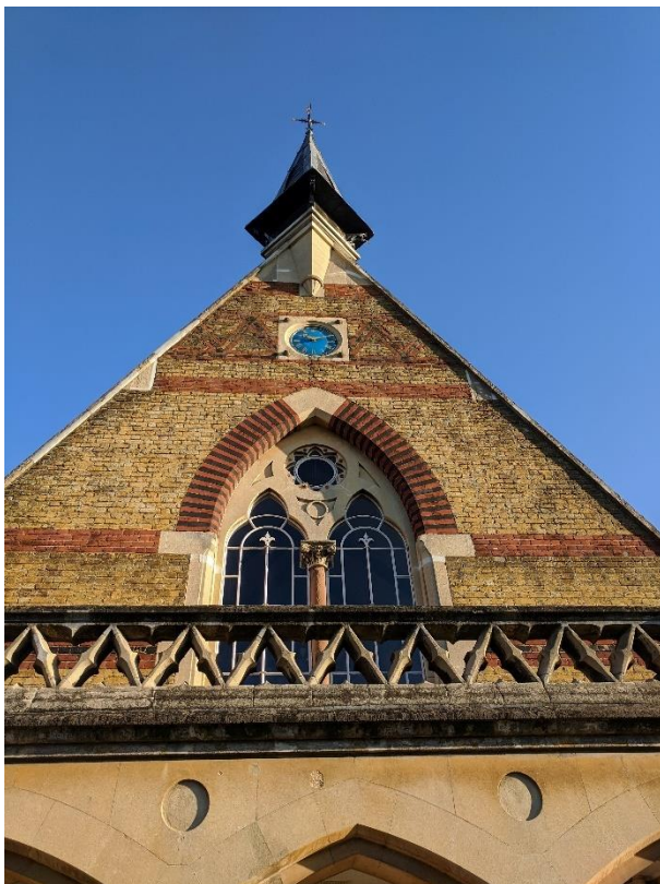
Photograph 8 - Front elevation of Chapel
