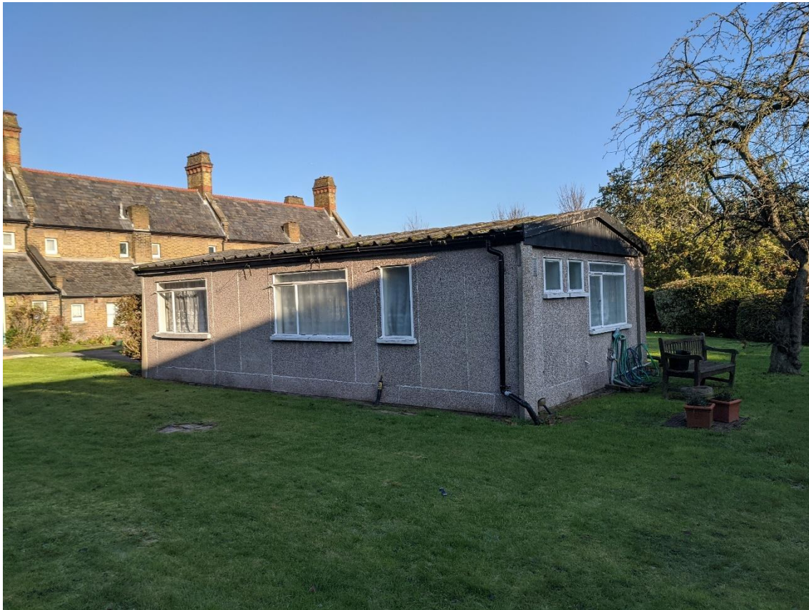
Photograph 9 - 1970's single storey laundry room
