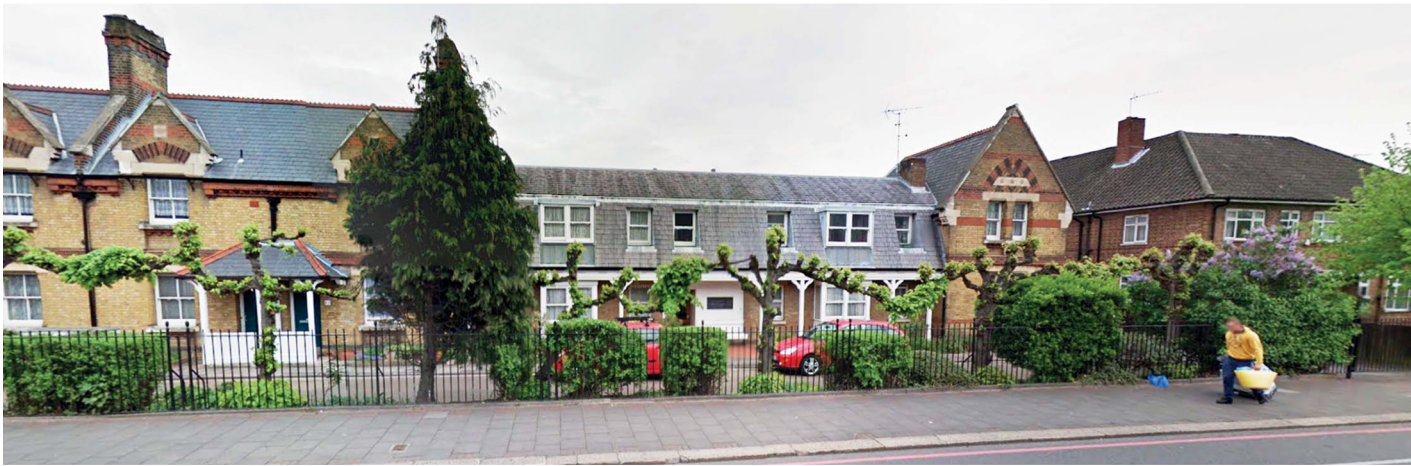
VIEW 2 - VIEW OF THE 1970'S INFILL BUILDING
