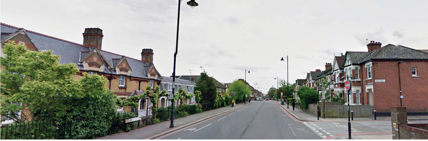
VIEW 6 - VIEW LOOKING SOUTH DOWN BRUCE GROVE
