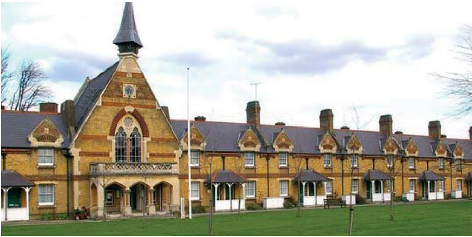
VIEW 1 - VIEW OF THE CENTRAL FORMER CHAPEL
