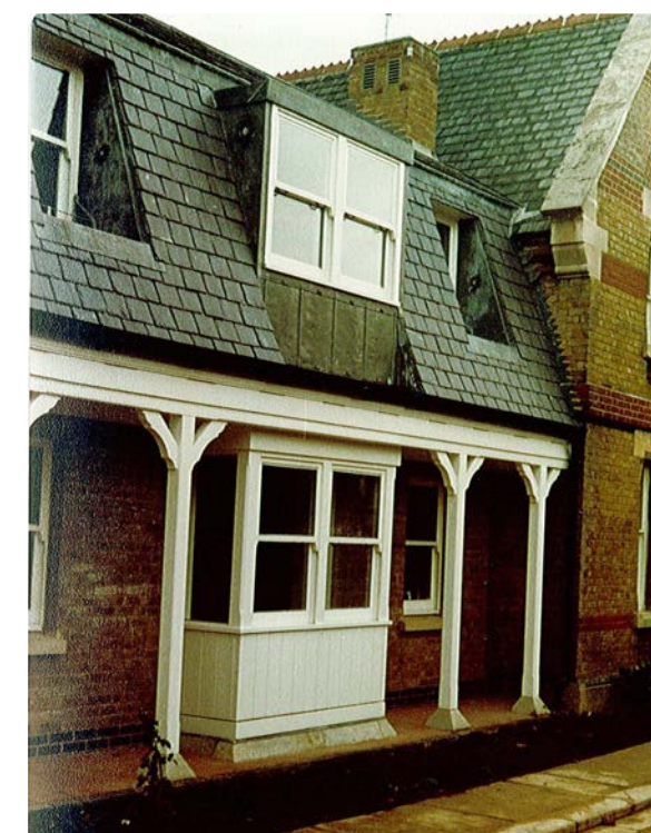
Figure 3.4 New infill between the Matron's Lodge and main Almshouse blocks designed by Berry Webber & Partners, architects and built 1978-1981. © Drapers' Company Archives.
