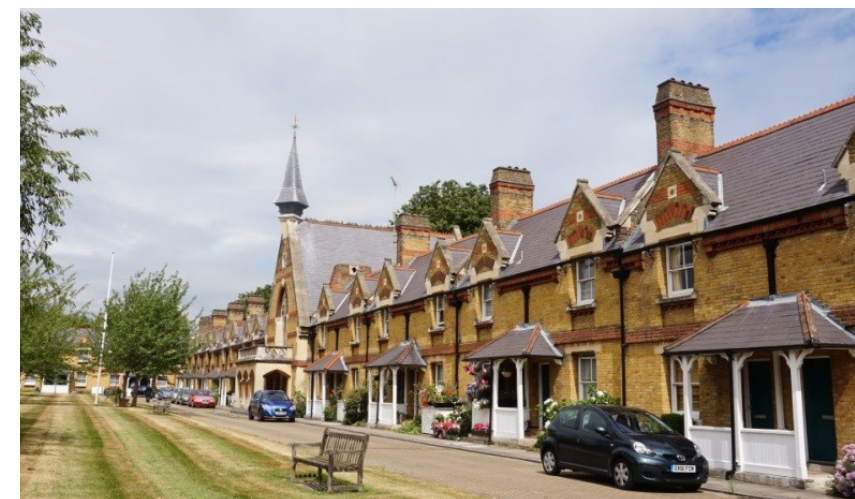
Figure 4.2. View of the Chapel and residential terraces.
