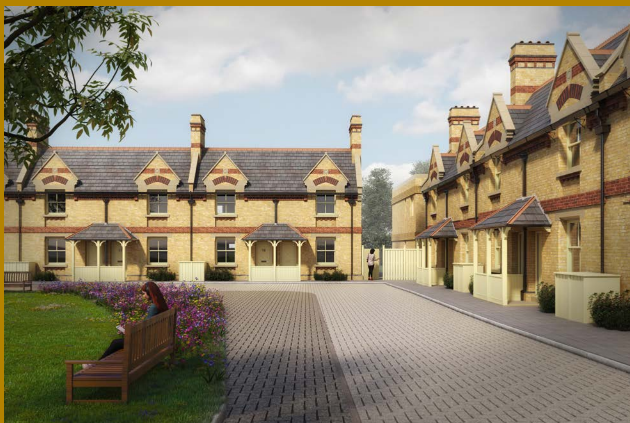
Figure 5.5. View from the roadway looking along the Almshouse towards the corner pavilions.
