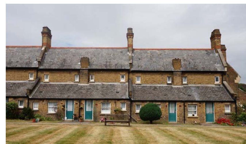
Figure 4.4. Rear elevation of almshouses.
