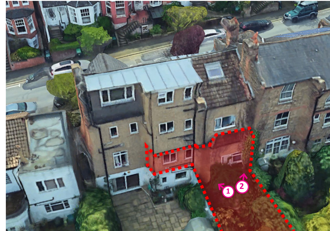
View of the rear elevation
