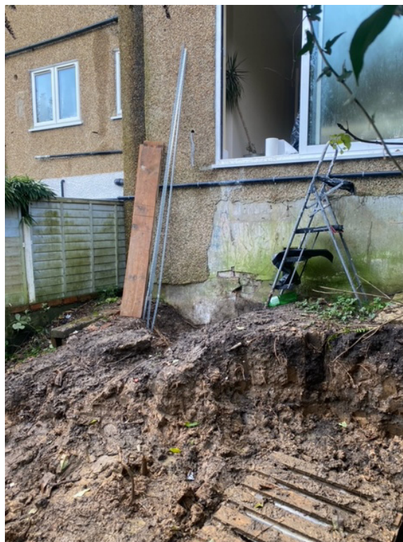
① Rear elevation & eastern boundary
