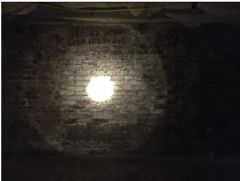
Blocked window below 26 central courtyard side. The arched brick head and the brick on edge cill of the original window are visible. All the basement windows below 24, 25 and 26 were blocked.
