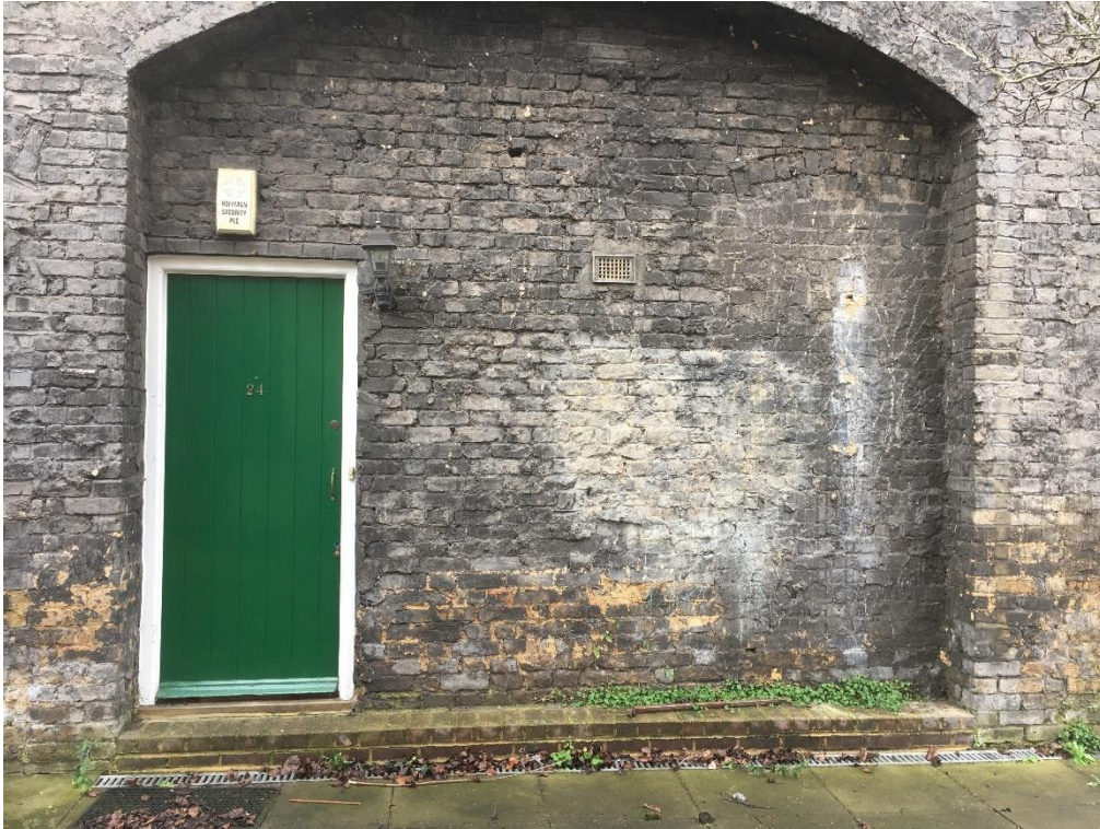
Wall to 24. The entrance door is set within brickwork that forms a recess from the principal wall face. The wall could be thin, 9 inches, because it originally was internal. All the brickwork has been painted with a grey colour-wash. The header arch to the right hand side is where there was a former door. Observe the plants at the raised brick upstand and the Acco drain at wall base. To the right and left of the door salt damage is causing disruption of the surfaces – a sign of bad rising damp.
