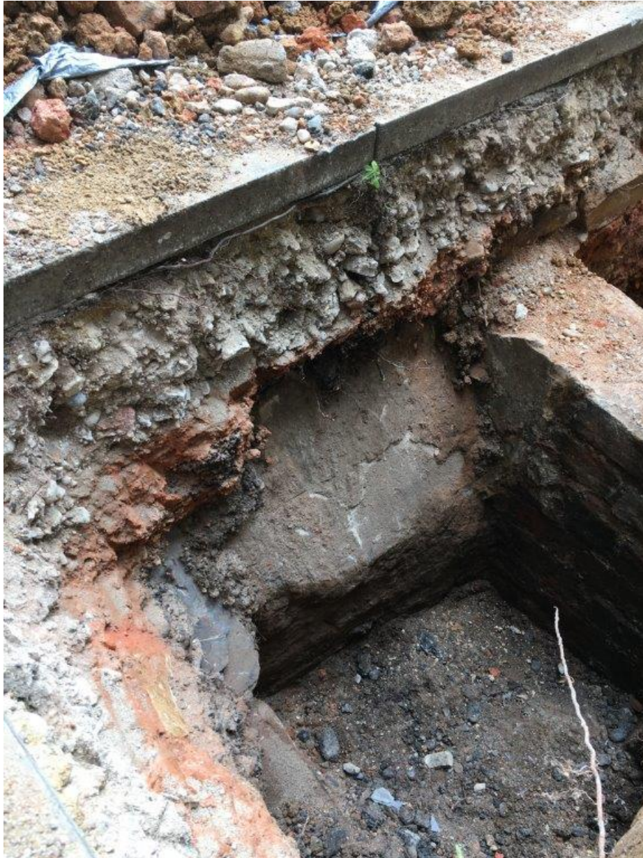
The top stone of the coal chute exposed.
