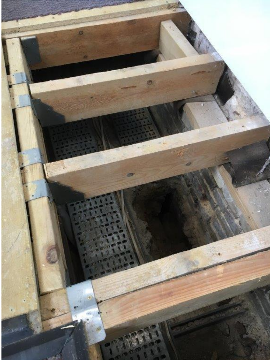
Recently constructed corridor floor structure
