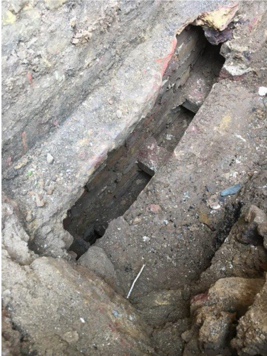
Pit 1. Detail showing the cavity constructed to guard against excessive wetting of the lower part of the external basement wall. This construction was found also at Pit 2 and at the front of the building at the external wall of Flat 3.
