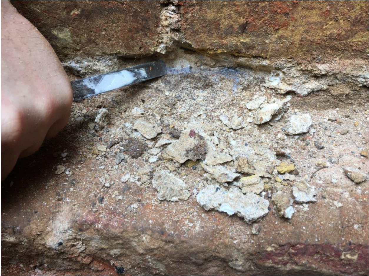
Original slate DPC exposed.
