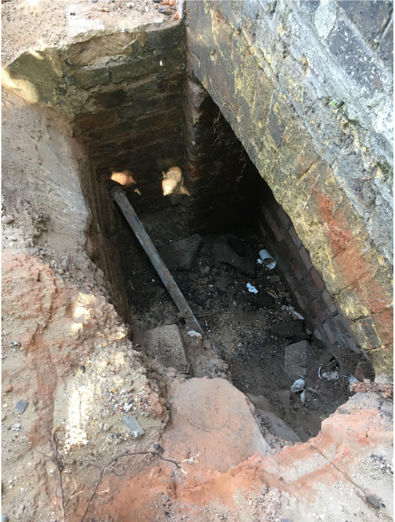
The extent of excavation at the basement “window” Flat 24.
