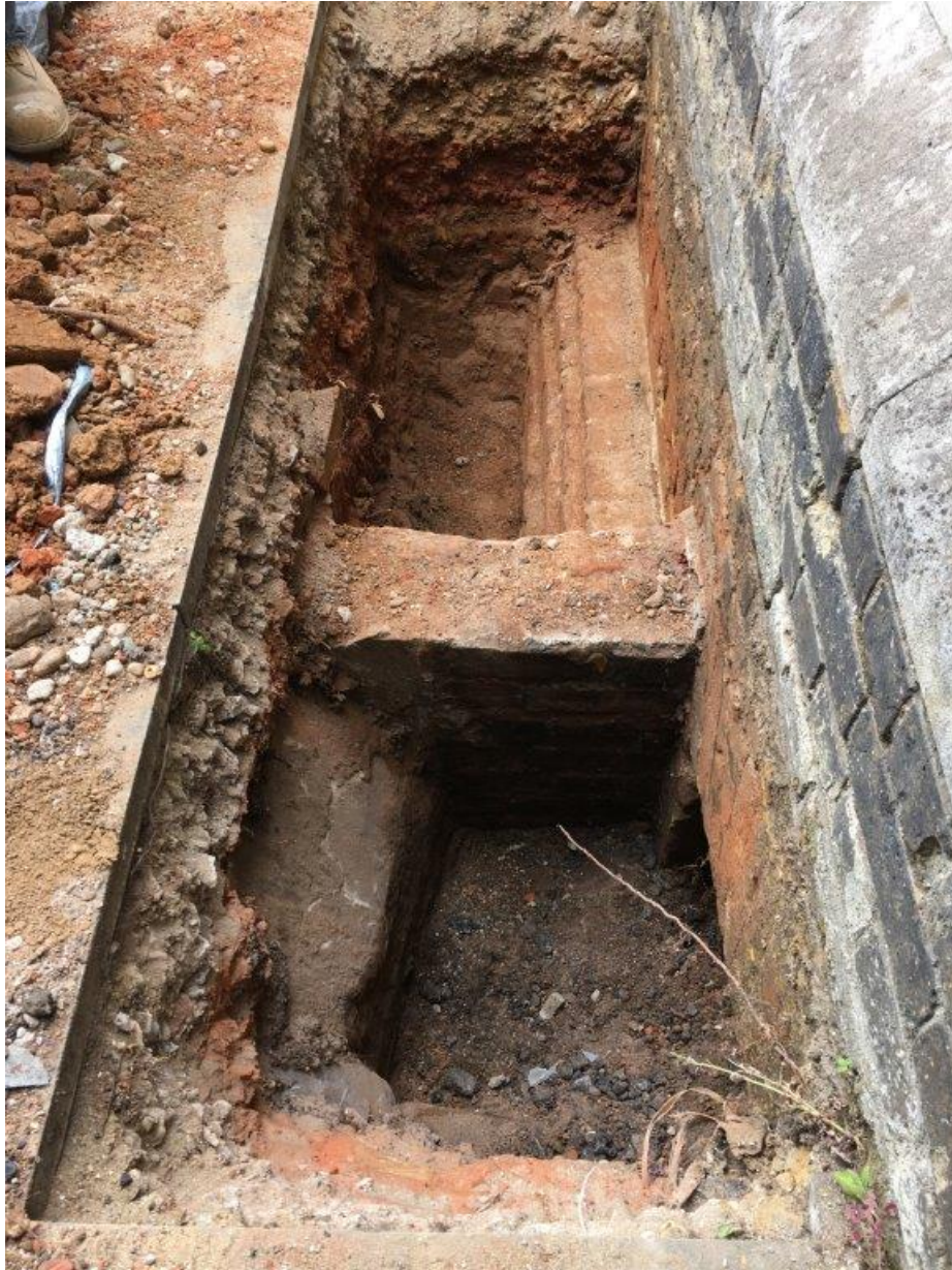
First stage excavation at Pit 2 exposing the top of the window arch (bottom of image), the vent area cross-wall and the brick set-offs denoting the external cavity construction.
