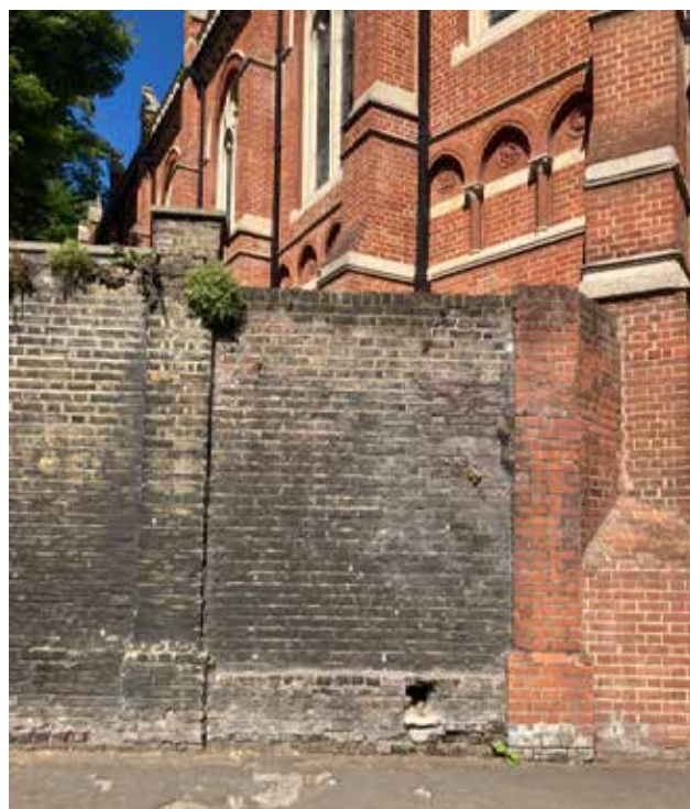
Figure 1.1. Photo of the wall abutting Highgate School Chapel
