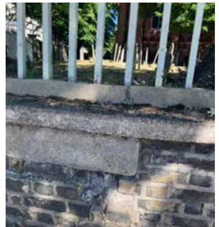
Figure 3.6. Concrete pad on top of coping
