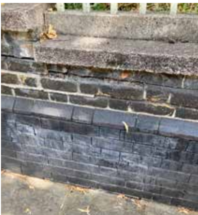
Figure 3.7. Layers of repair to wall
