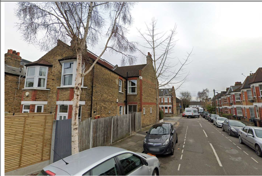
Photo 1 – View of side and rear of No. 36 Kirkstall Avenue N17 6PH. [Source – Google Maps 2022]
