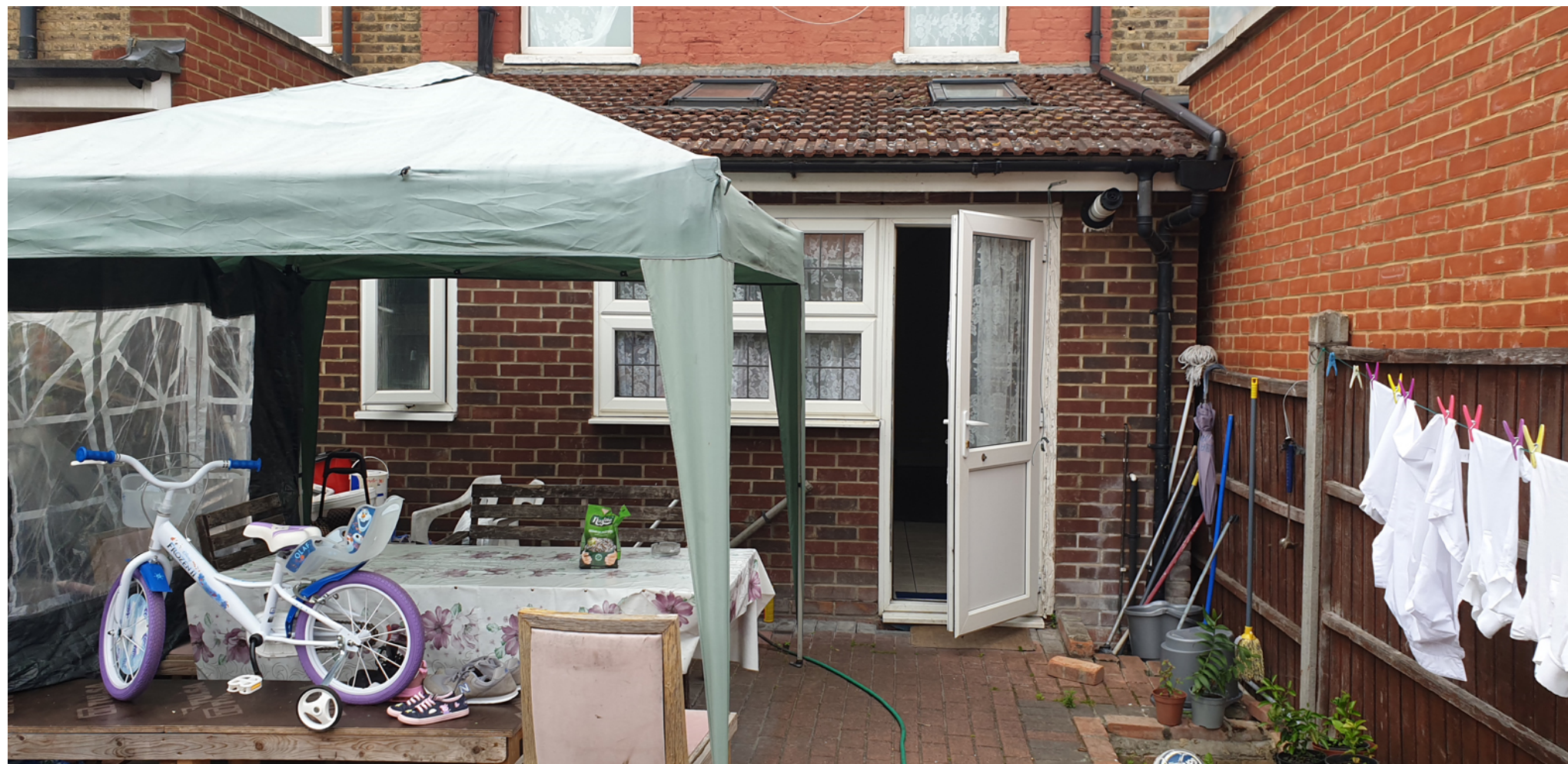
Application Site - Rear Elevation - Ground Floor
