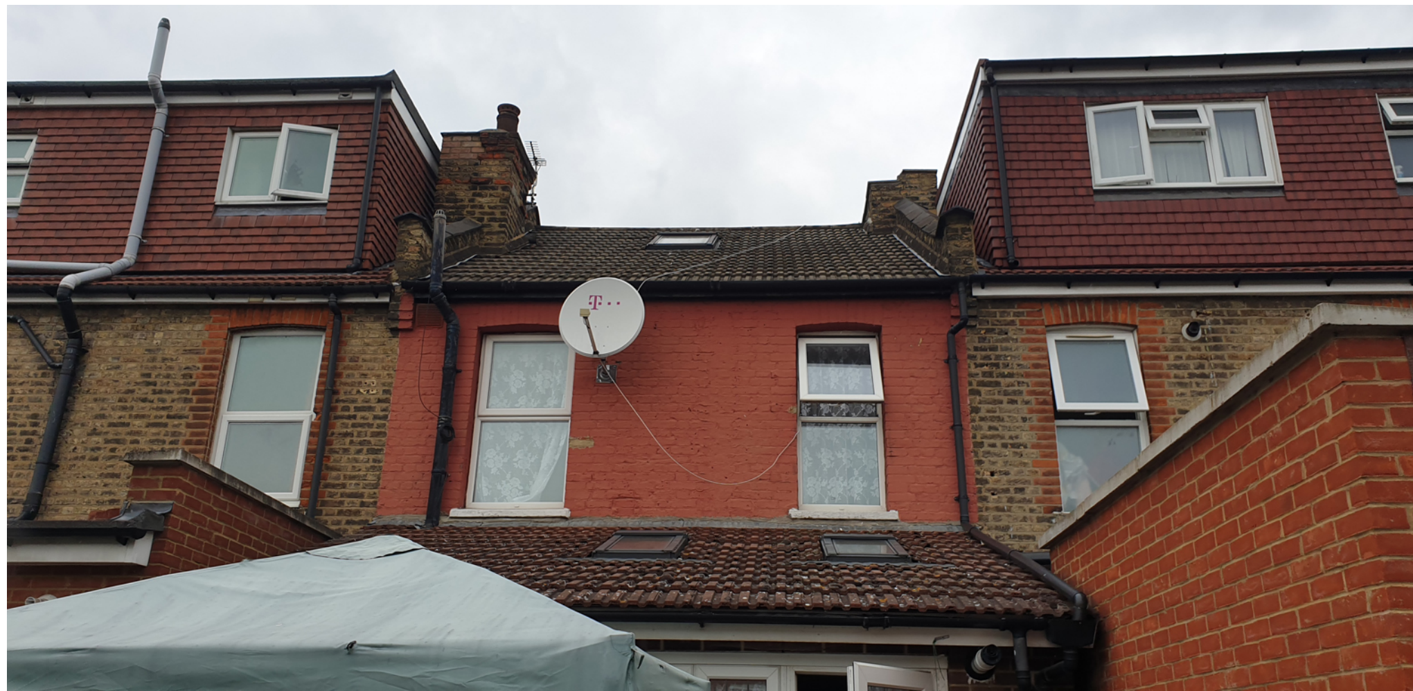
Application Site - Rear Elevation - First Floor
