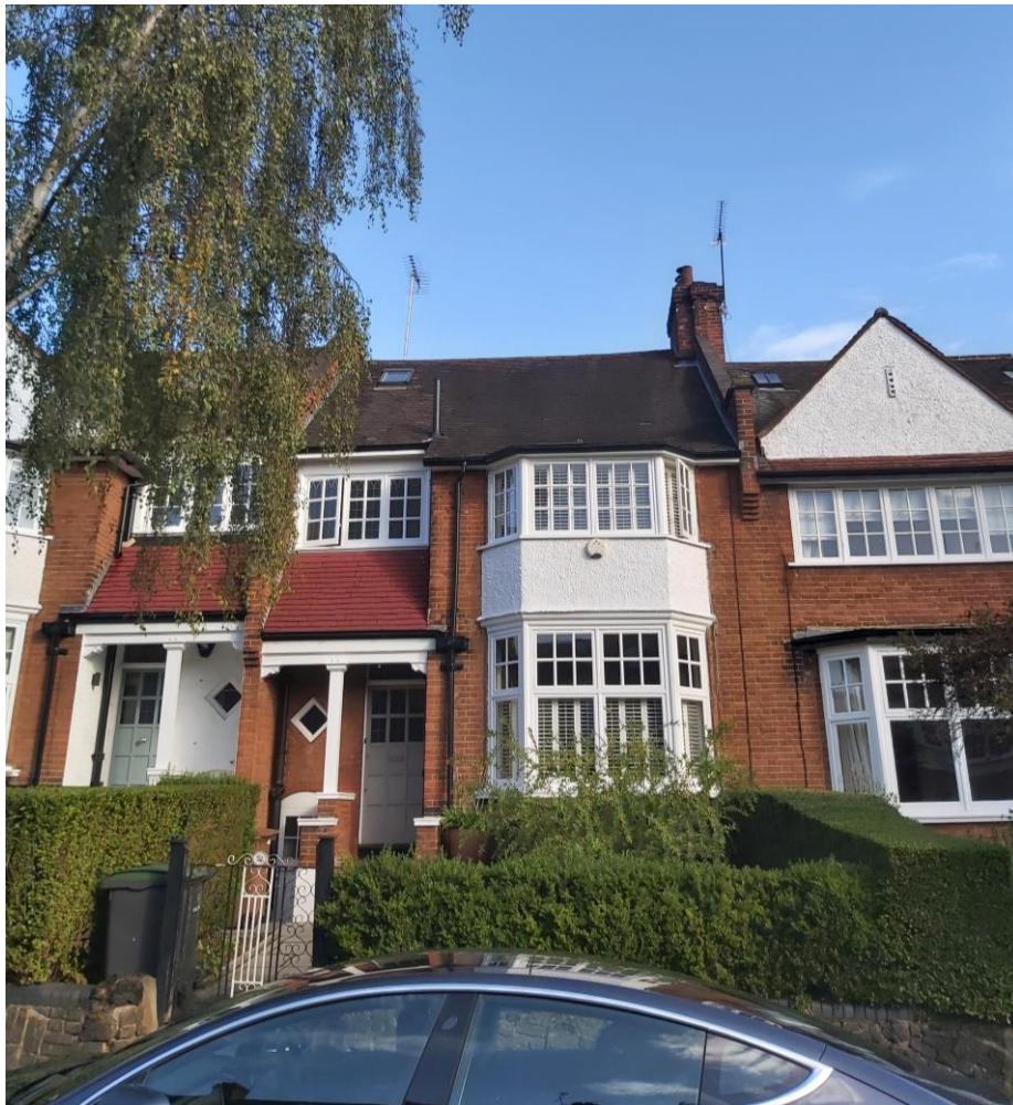
Fig.1 Photo showing front elevation of existing property
