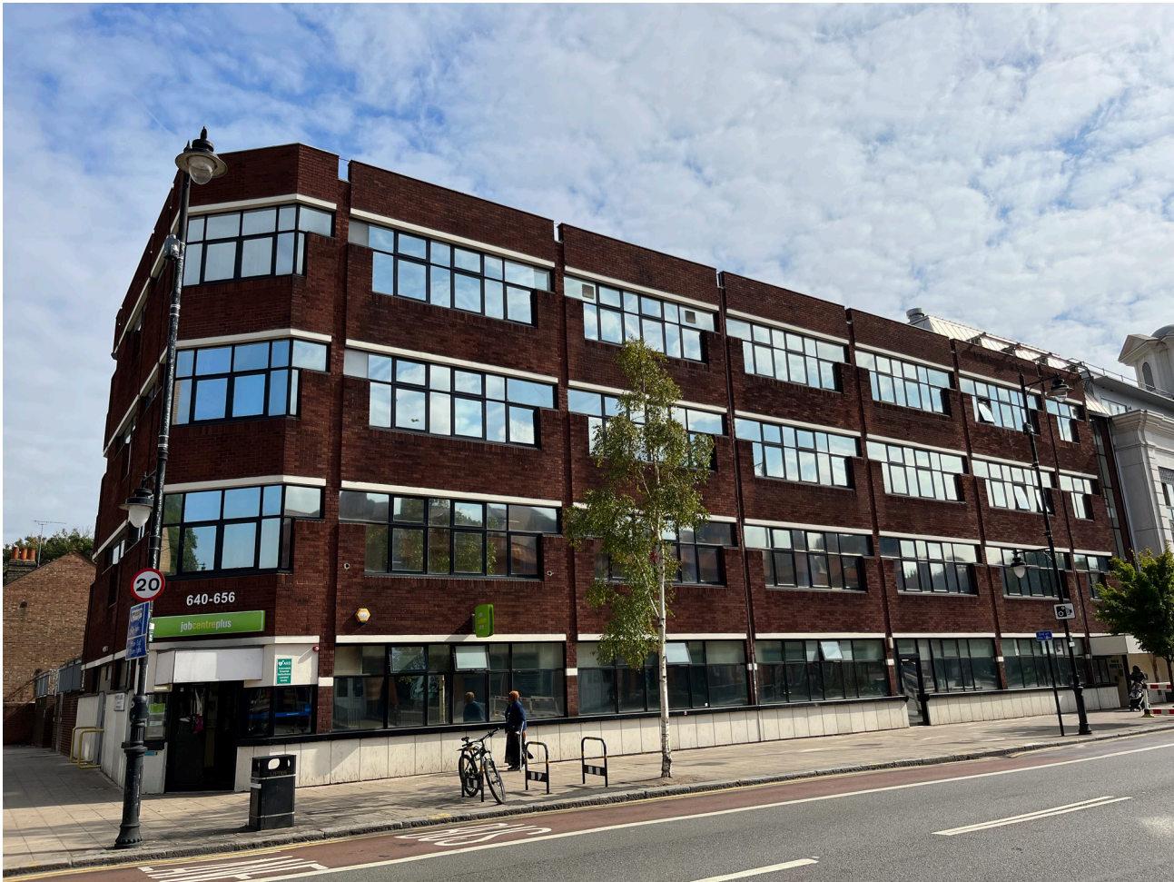
View of the existing building
