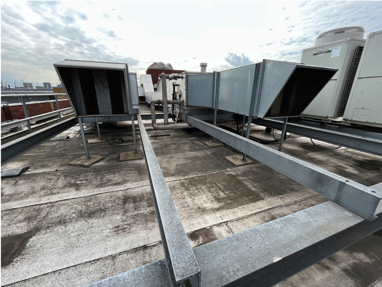
View of the existing plant on roof
