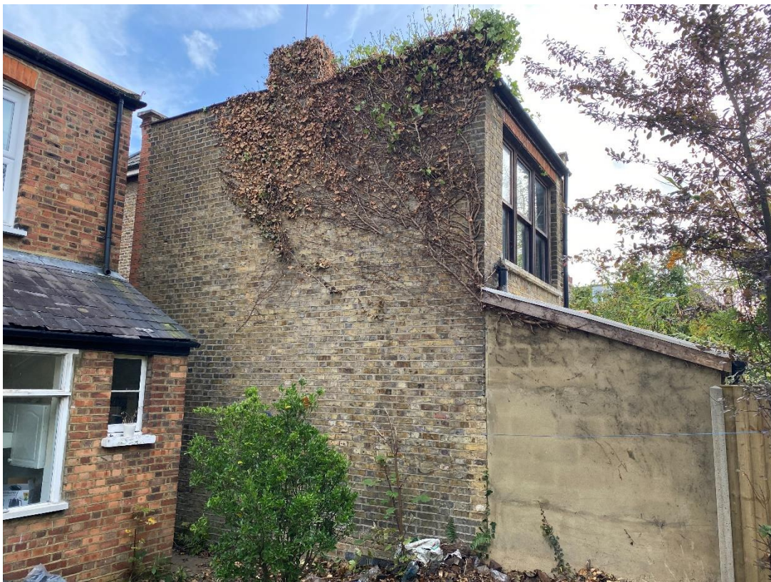
Photo 8: Flank wall and extended rear building line at No.1 Curzon Road
