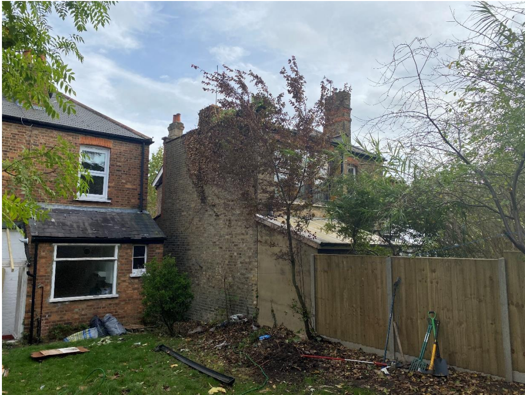
Photo 7: Rear of No.3 Curzon Road with flank wall and set-back building line of No.1
