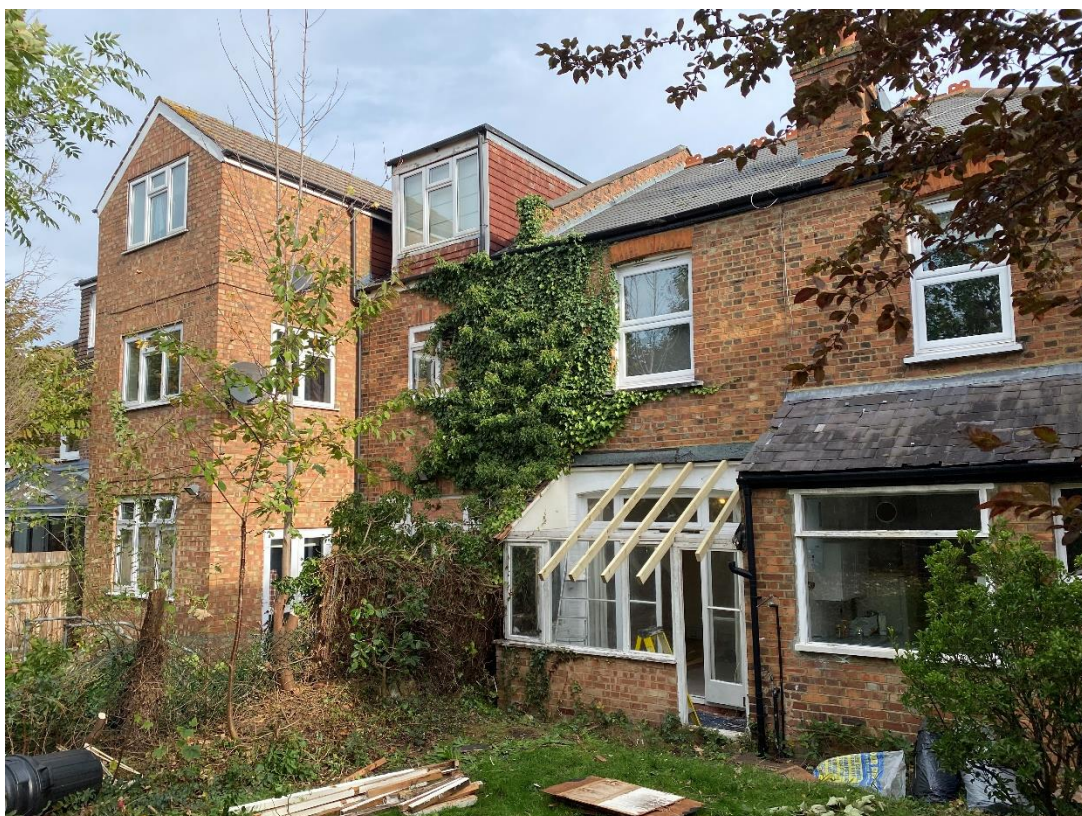
Photo 3: Rear of No. 5 Curzon Road, with 3 storey extension
