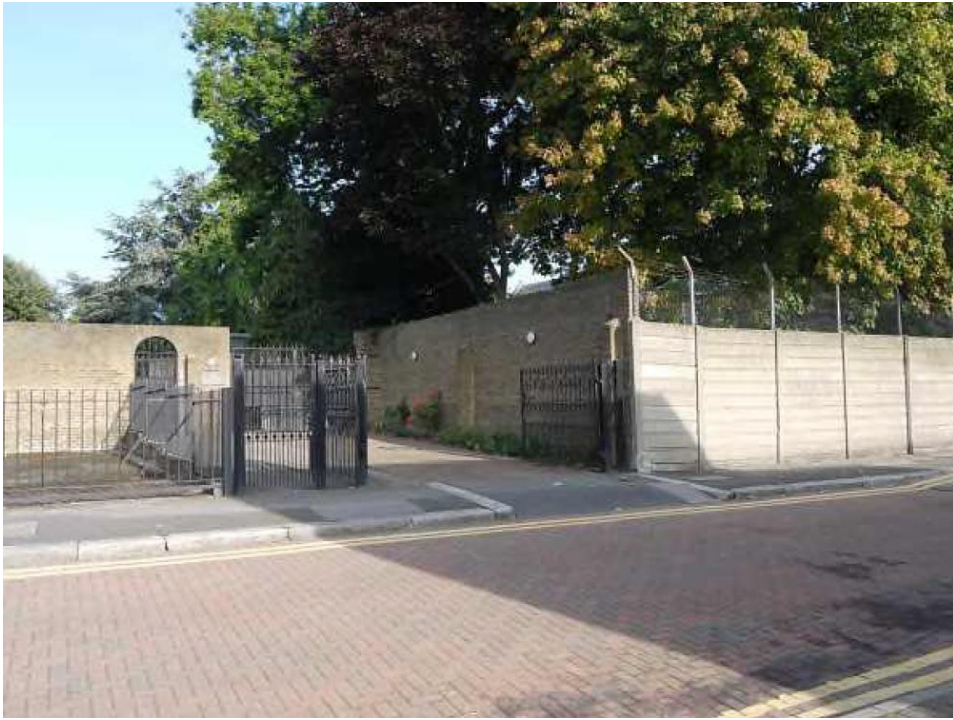
Photo No.12: View to north-west of boundary wall surrounding mosque garden from Suffolk Road
