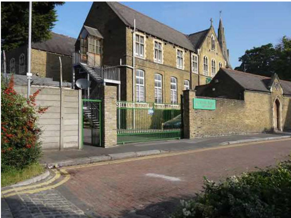
Photo No.8: View of pedestrian and vehicular access to private school off Suffolk Road, view to west
