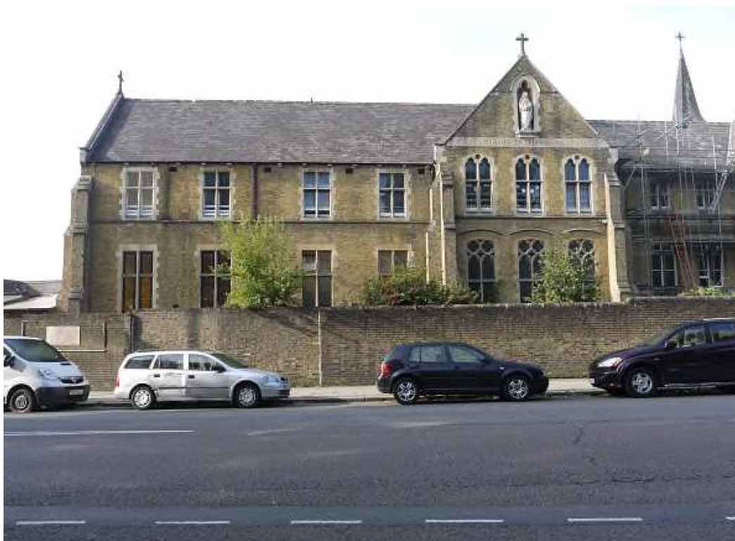
Photo No.2: Northern elevation of Old Priory Buildings and boundary wall from St Ann's Road
