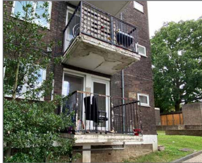
South West facing balconies
