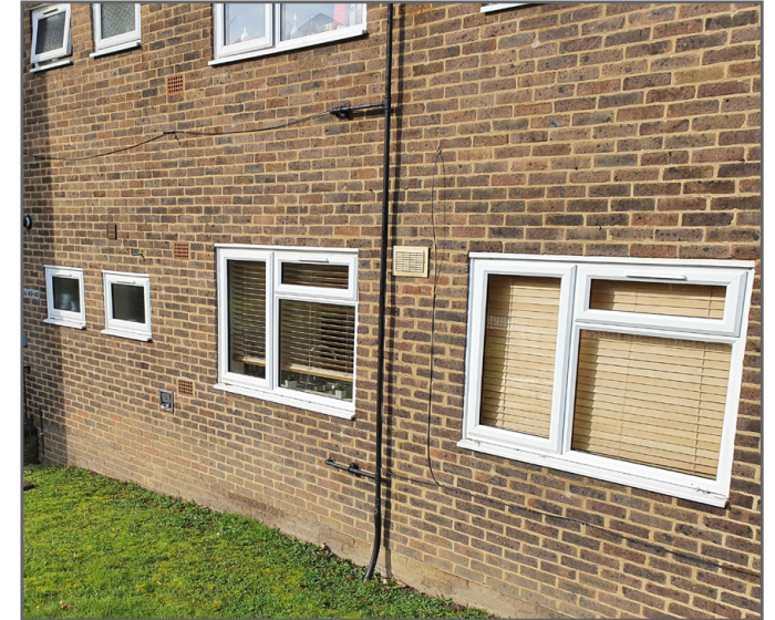
White PVC windows within brickwork facade
