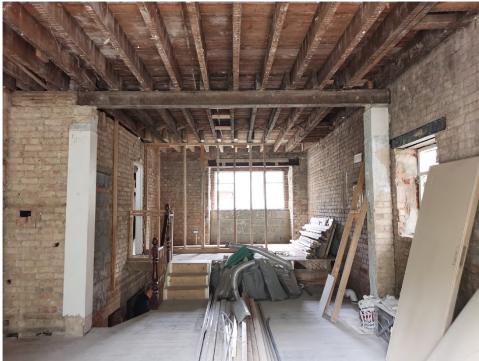
Photo 3 – Ground Floor looking towards the rear
