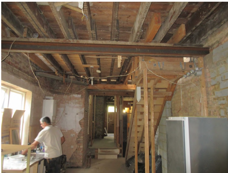
Photo 4 – Ground Floor looking down the hallway to the front
