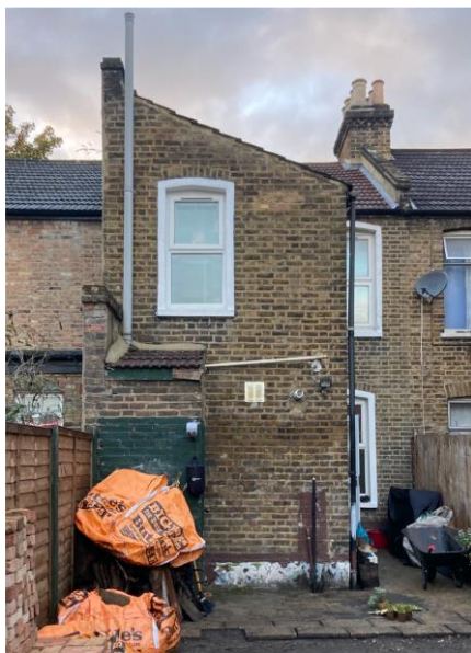
Photo of rear elevation
