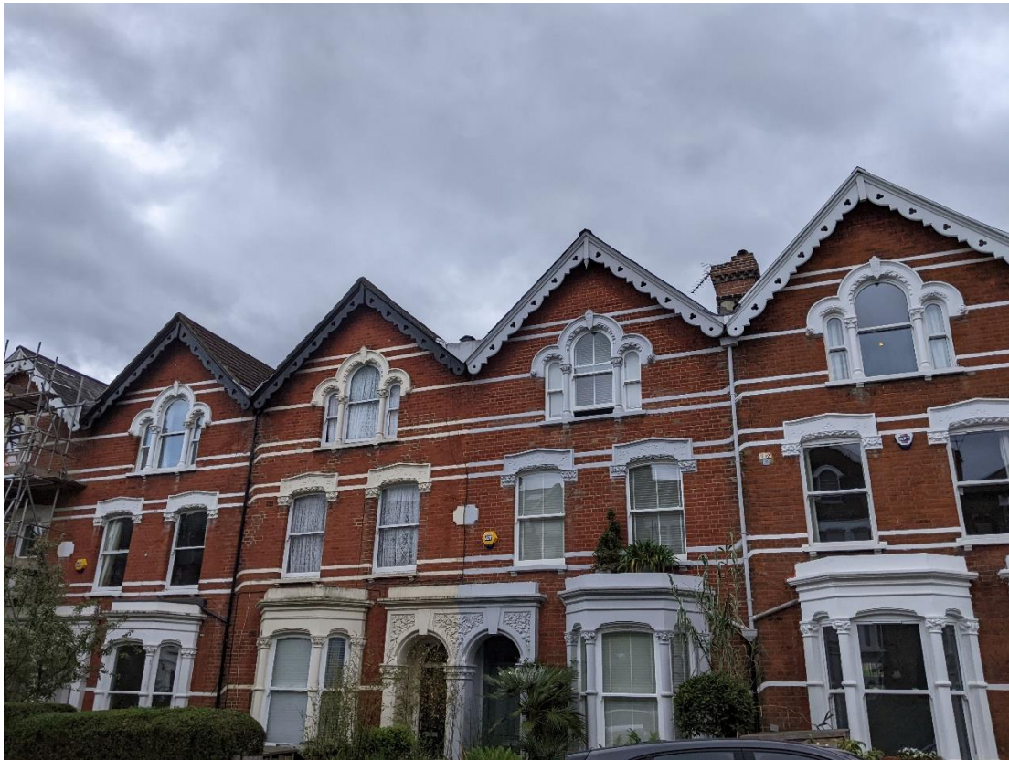
Figure 1: Front elevation of the terrace. The site is located on the left hand side next to the scaffolded property at no.86.
