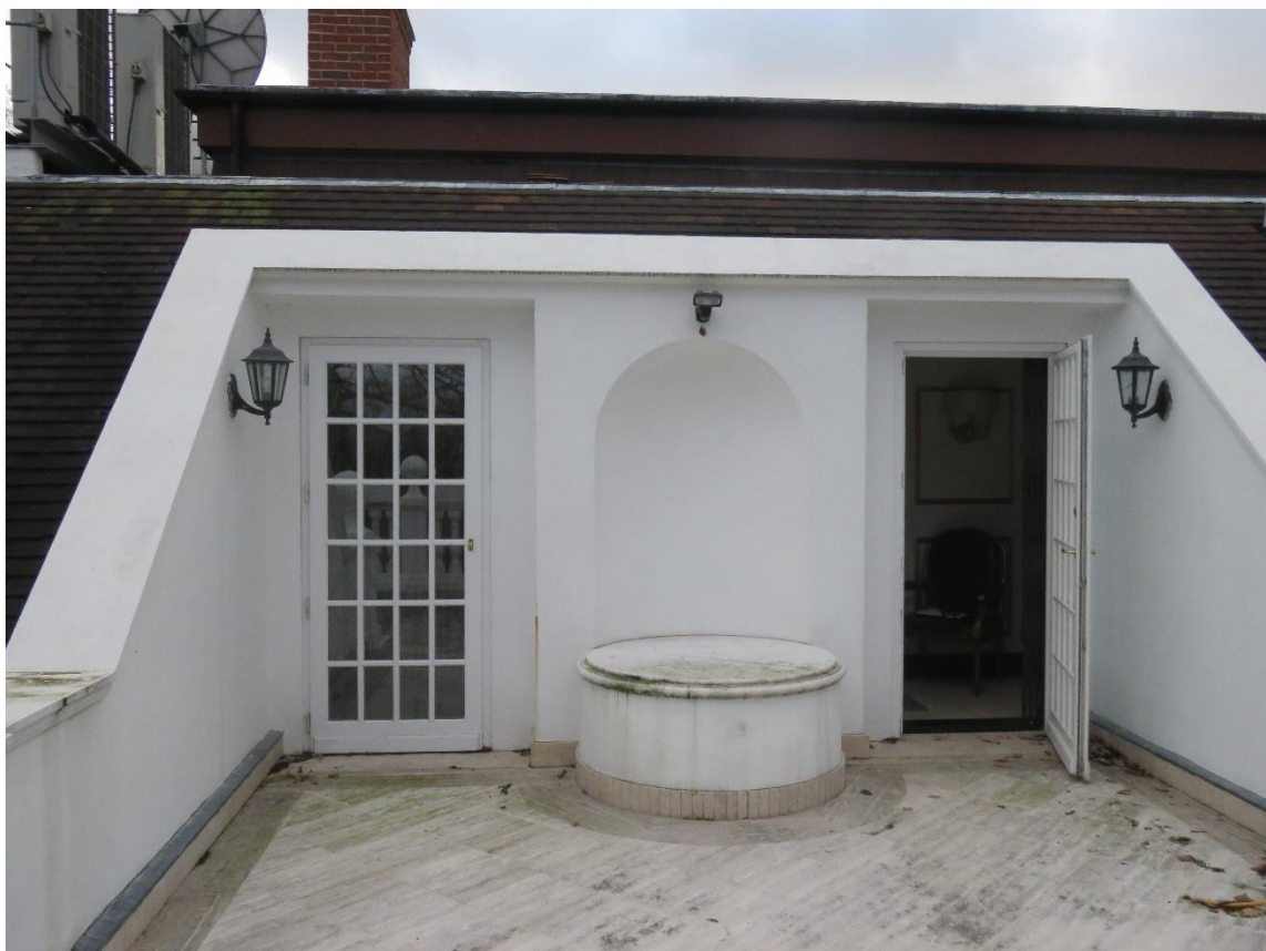
Above images: Views of the existing northern side roof terrace which is proposed to be replaced with an extension to the main pitched roof.
