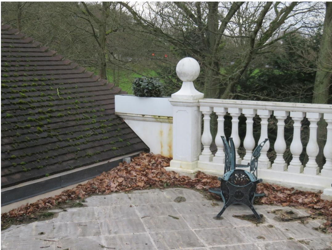
Above images: Views of the existing northern side roof terrace which is proposed to be replaced with an extension to the main pitched roof. It is proposed to remove the stone bottle balustrading.
