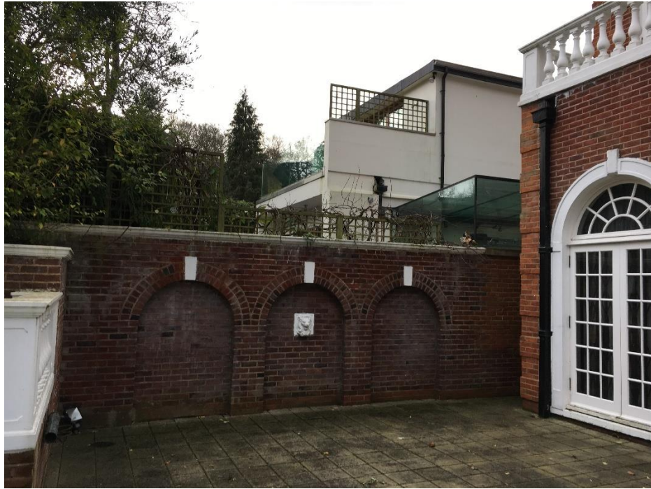
Above: View of the south boundary wall to the site taken from the rear garden.
