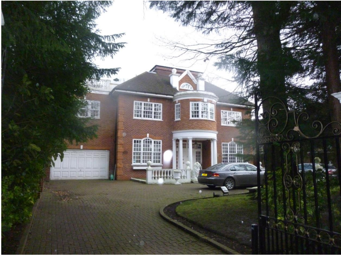
Above: the application site viewed from the entranceway on Courtenay Avenue
