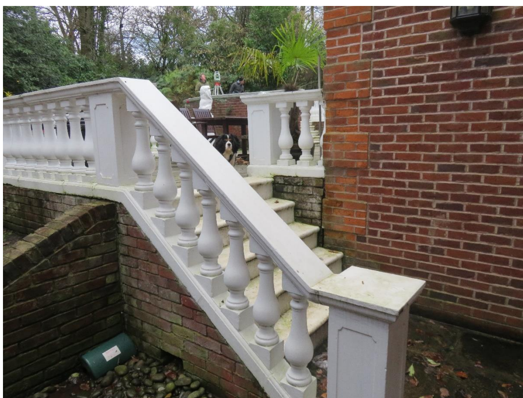
Above: View of the north side of the property at the rear of the existing property showing the changes in level.
