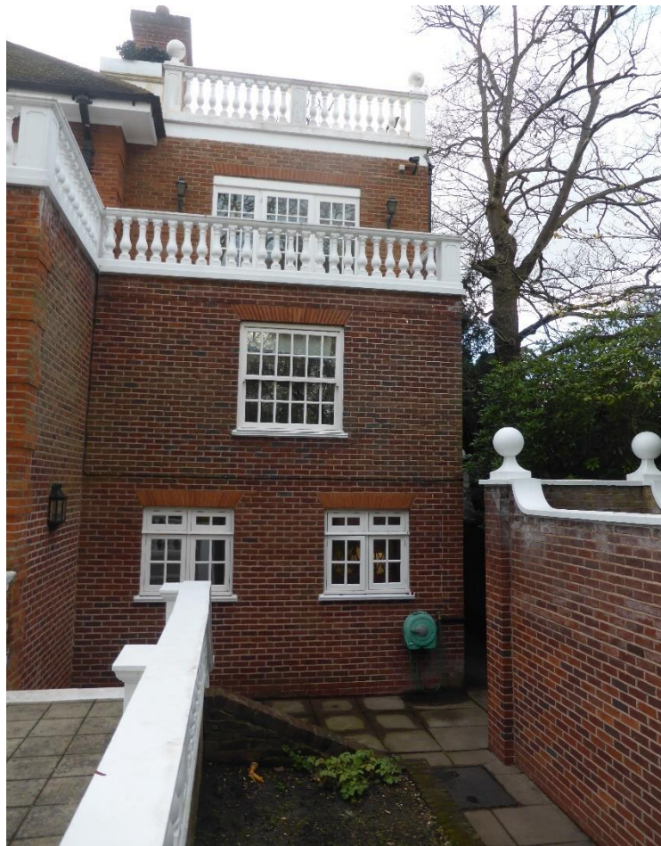
Above: View of the north boundary wall to the site taken from the rear garden. The changes in level can be seen with stepped access.
