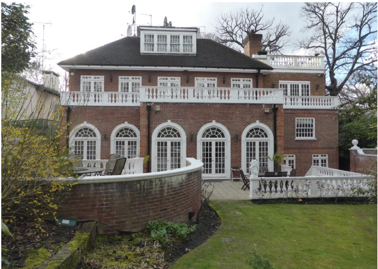
Above: View of the rear of the existing property
