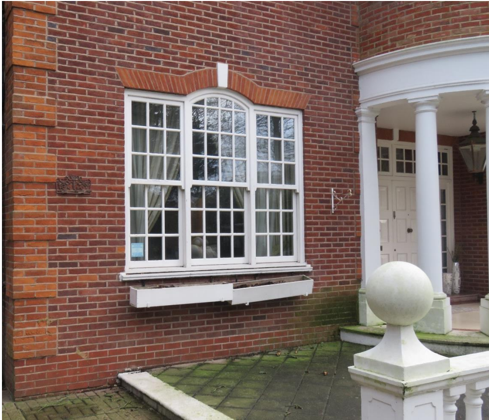
Above: the existing front elevation showing the brick quoining detail and brick plinth. These details will be replicated in the new build extensions at the rear of the property, ensuring a cohesive design throughout.
