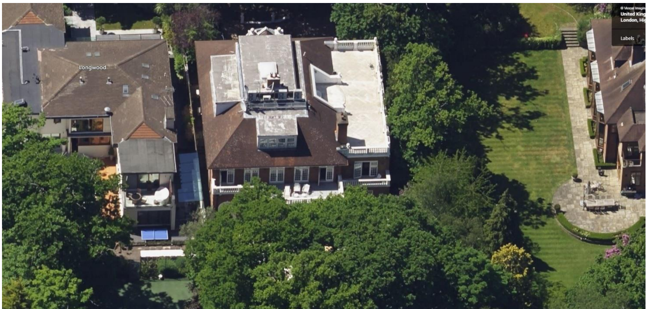
Above: East facing Birdseye view of the site (rear elevation)
