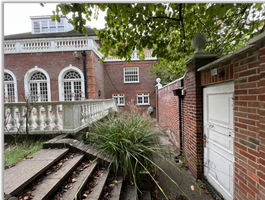
View of Rear of Building and Outbuilding
