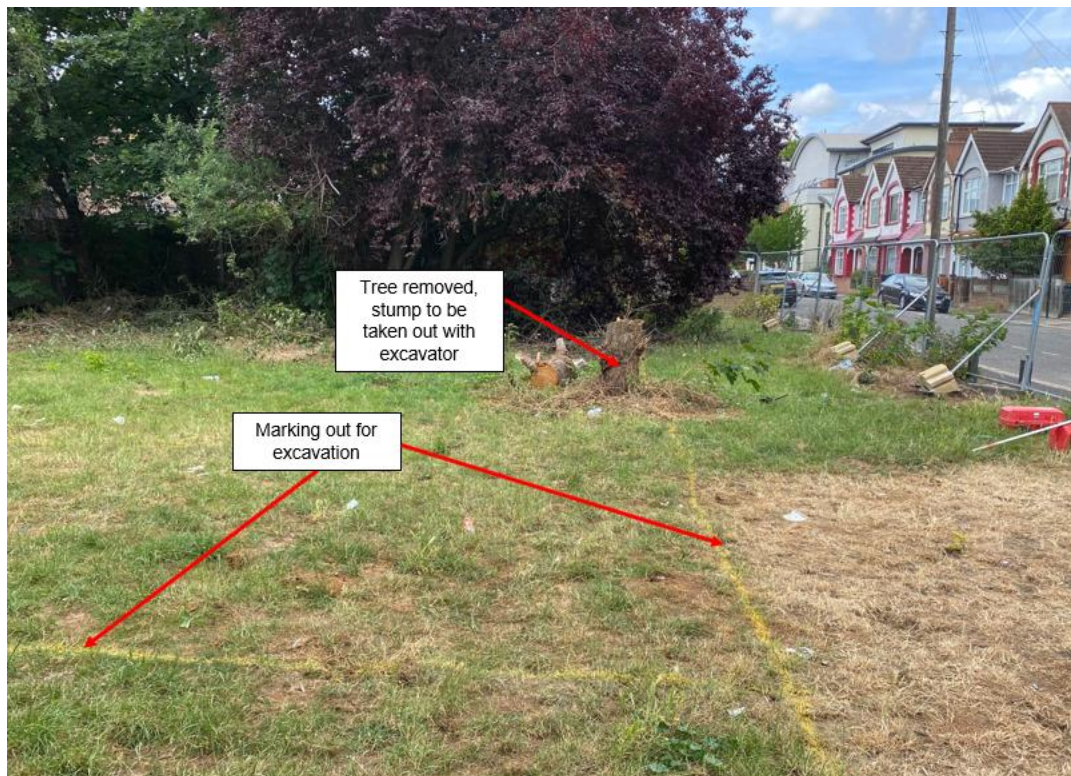
Looking west across park area showing setting out for new slab
