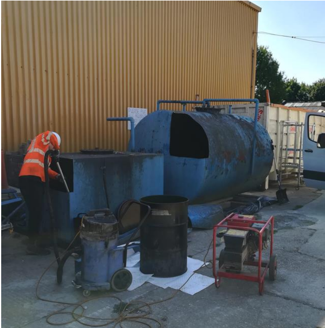
Tanks being cleaned prior to removal from site for re-cycling of the steelwork.
