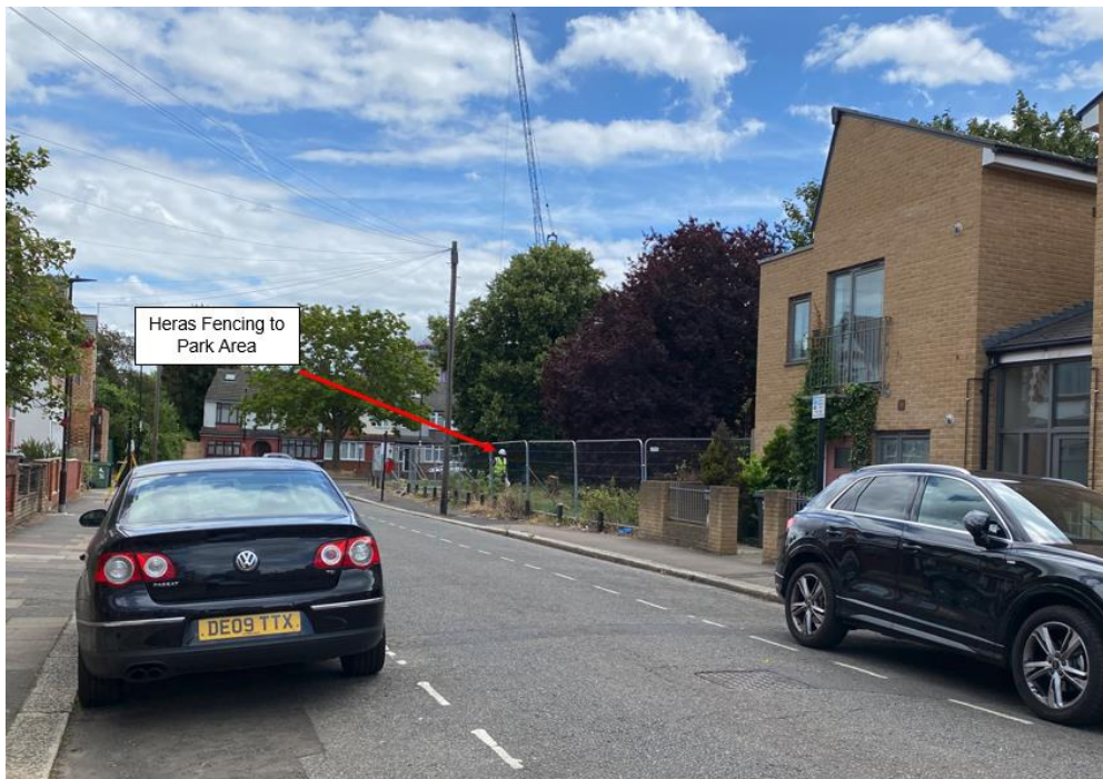
Park area fenced off to allow erection of hoardings and site works to commence
