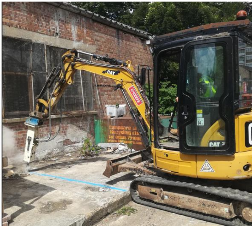
Demolition Works to Concrete slabs in Yard - commenced
