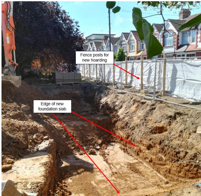
Looking west across park area showing excavation for new slab
