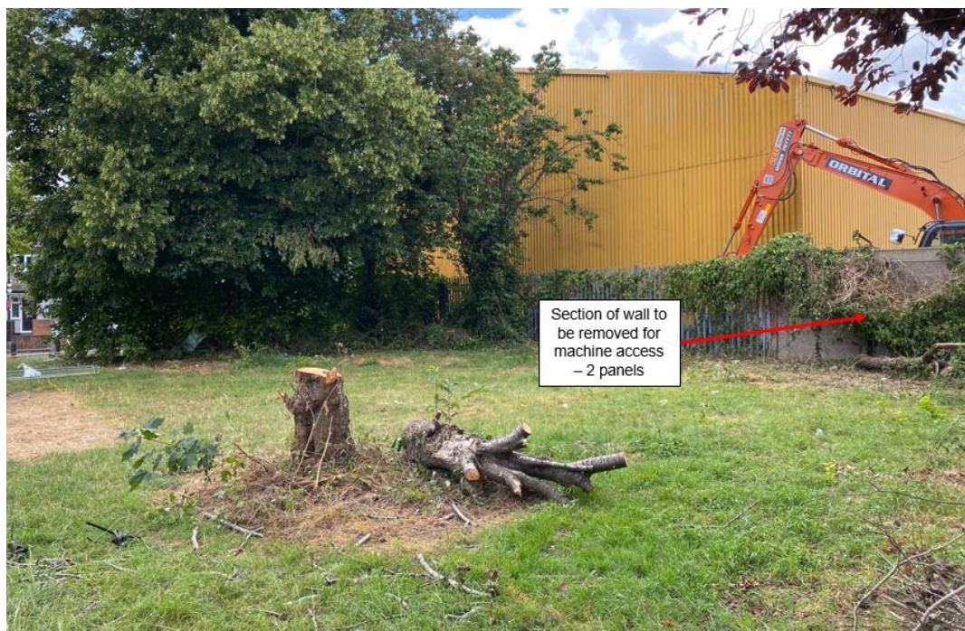
Looking east across site showing cleared area and excavator
