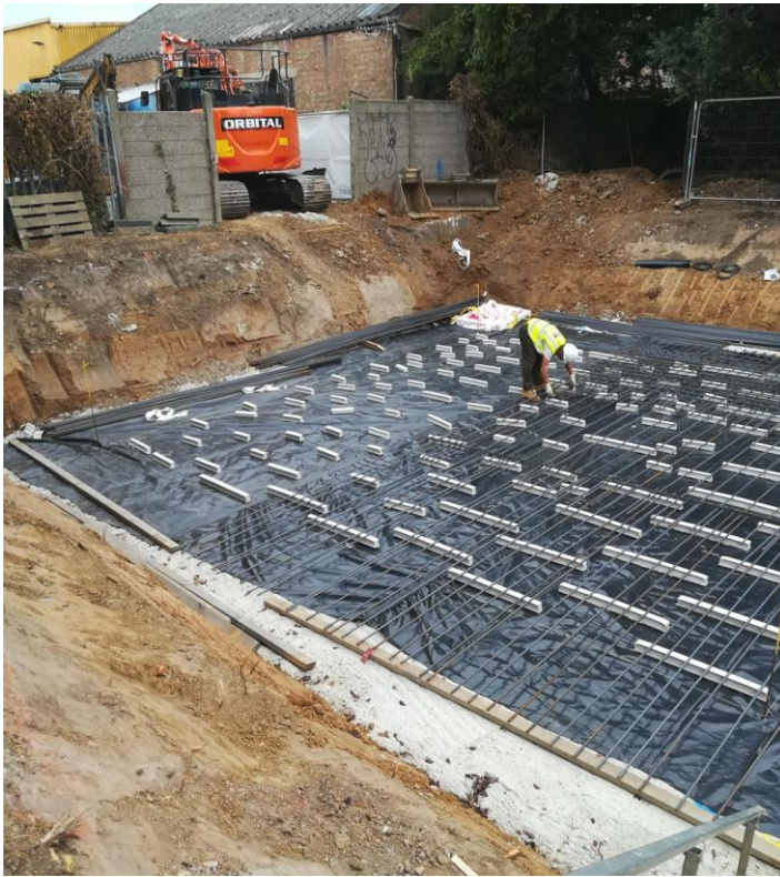
Excavation complete, rebar being fixed, waterproof membrane in place (excavator in view)
