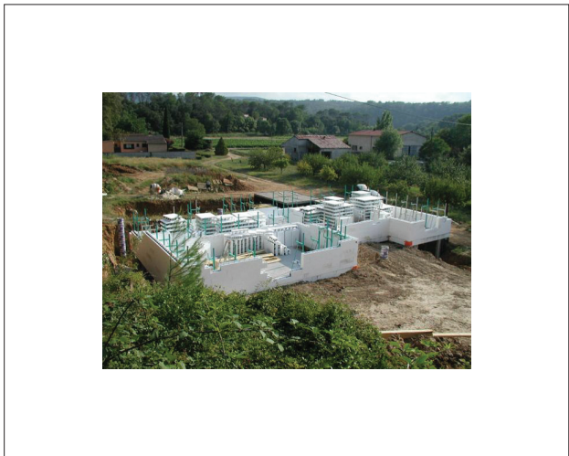
Figure 4 Construction site with trestles
