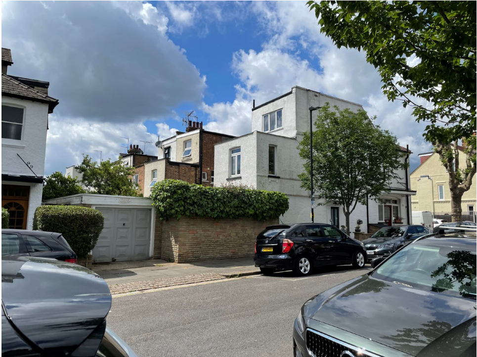
View of the rear elevation and view of the rear of the adjacent terrace
