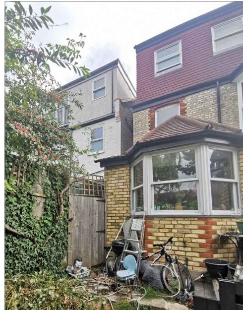
Rear elevation towards number 28
