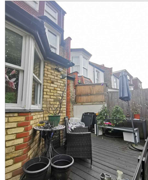
Rear elevation towards number 32
