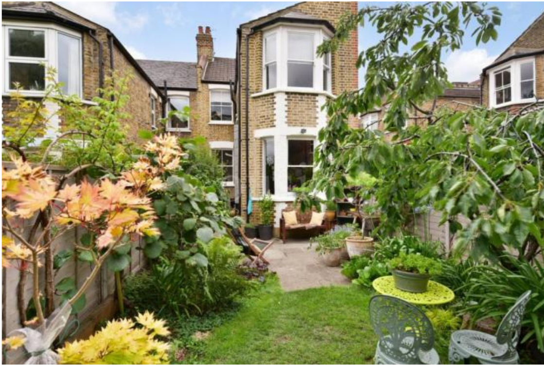
Rear elevation view of No.24 (left) and No.26 (right) Ripon Road
