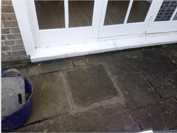
Fig 2.1: Trial Hole 2 Location
