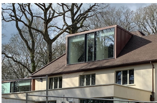
Examples of well-proportioned and carefully detailed zinc sheet clad dormers by ZDB Architects
