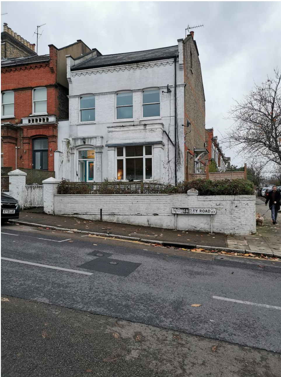
Front of the property from Womersley Rd
