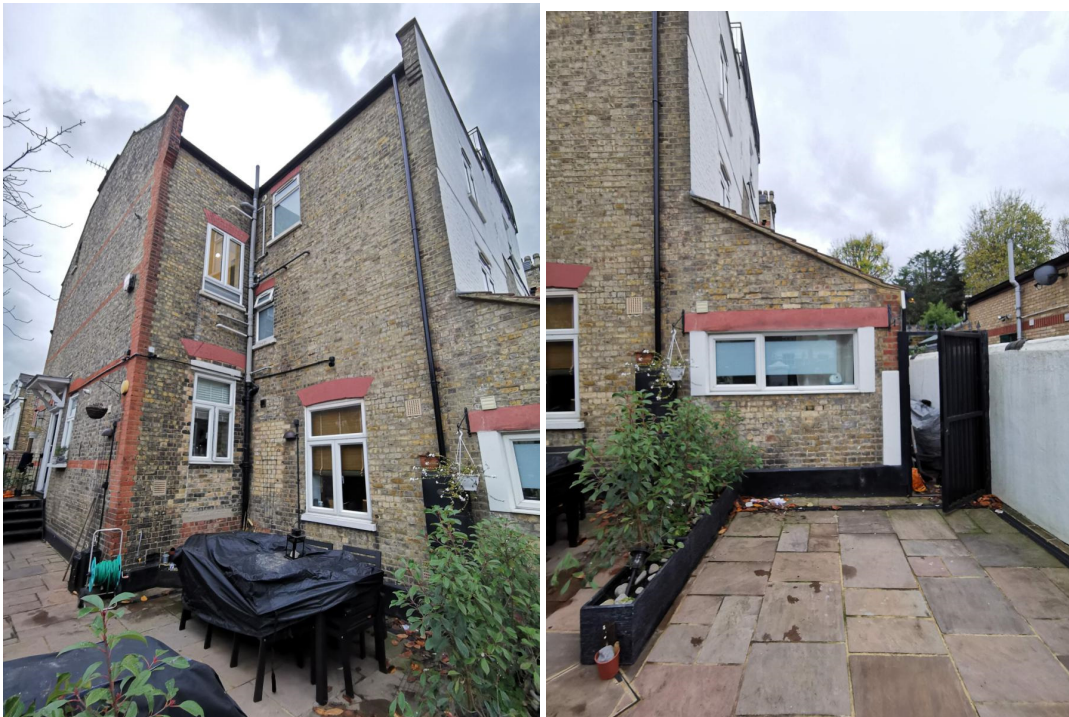
Rear of property from garden
