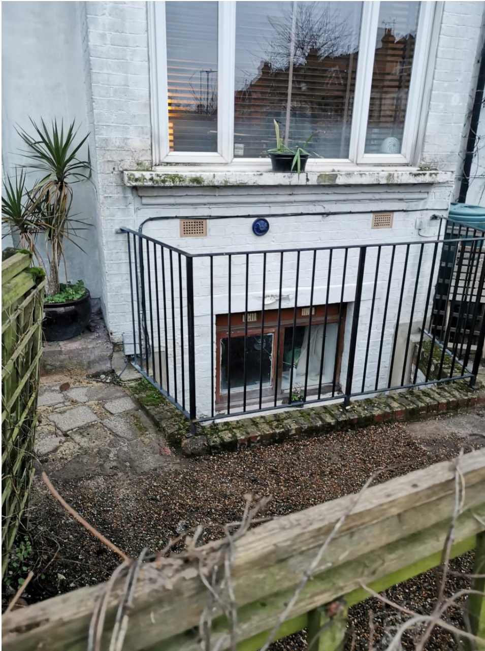
Existing light well to the front of the property
