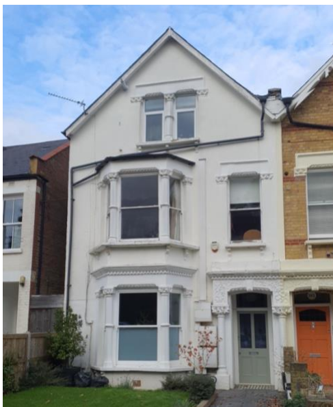
Front elevation of main property
