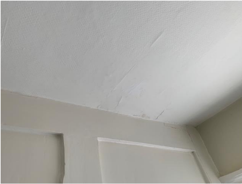
Pic 10) internal from front valley directly underneath pic 9
