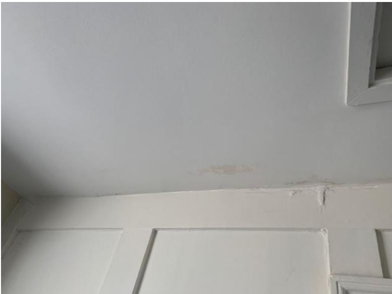
Pic 11) opposite side of the internal timber paneling pic 10
