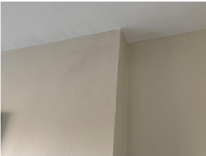
Pic 13) side wall of rear adjoining neighbor
