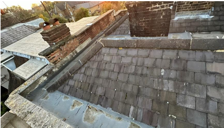
Pic 6) front picture of the two pitched roofs
