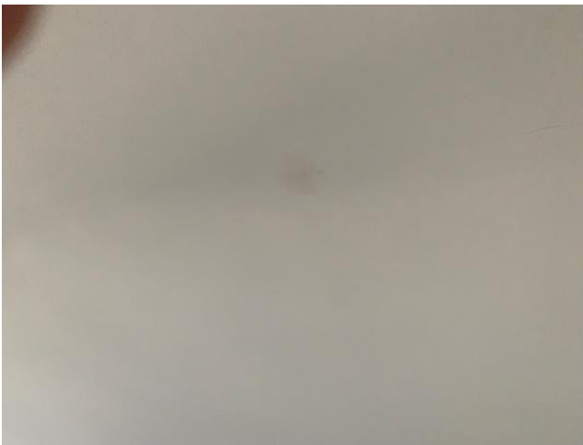
Pic 14) ceiling of rear room under the pitch roof
