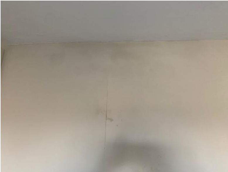
Pic 12) spine wall central to center valley
