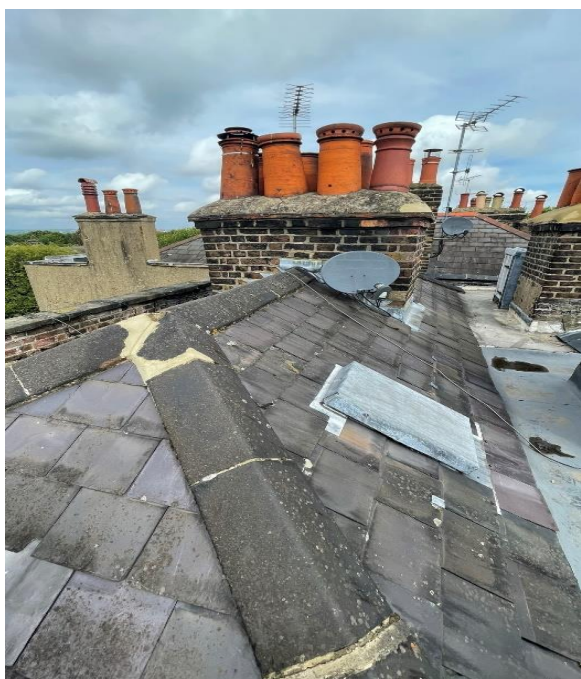
Pic 7) cement repairs to ridges
