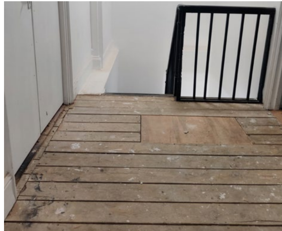
FIGURE 19. 792-G-02 Existing Floorboards
