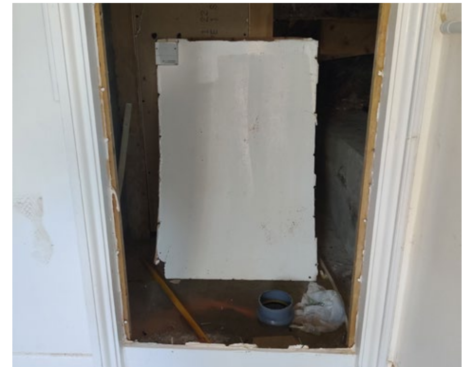
FIGURE 52. 794-B-06 Existing Cupboard
