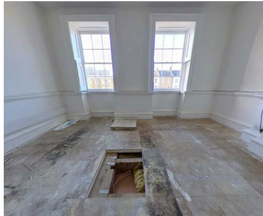
FIGURE 25. 792-F-04 No Evidence Of Floorboards
