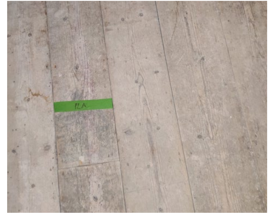
FIGURE 30. 794-F-07 Existing Floor Finish To Be Retained
