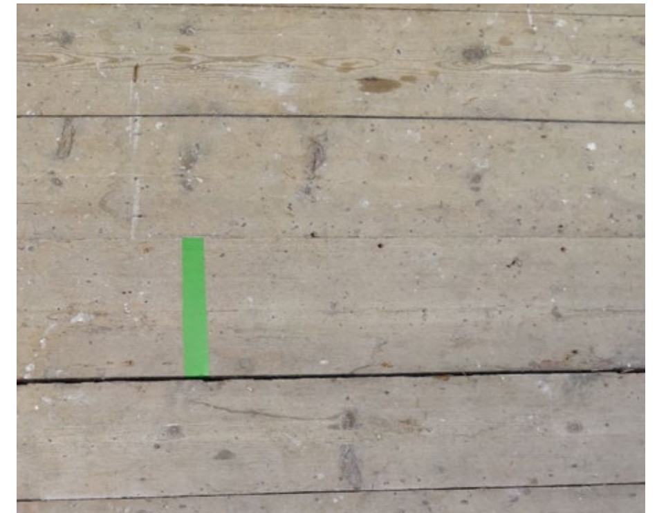
FIGURE 24. 794-G-06 Existing Floorboards demarcated to allow for opening up
