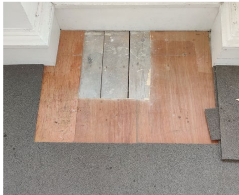
FIGURE 20. 792-G-04 Existing Floorboards visible through following removal of modern finishes
