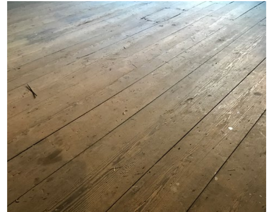
FIGURE 23. 794-G-03 Existing Floorboards in good condition
