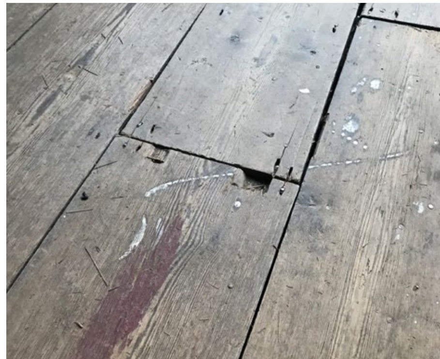
FIGURE 22. 794-G-04 Existing Paint Marks and spliced ends
