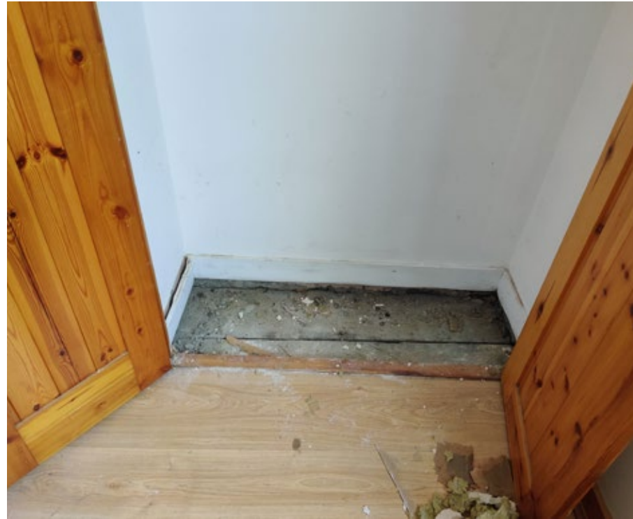
FIGURE 35. 794-S-03 Existing Floor Finish To Be Retained
