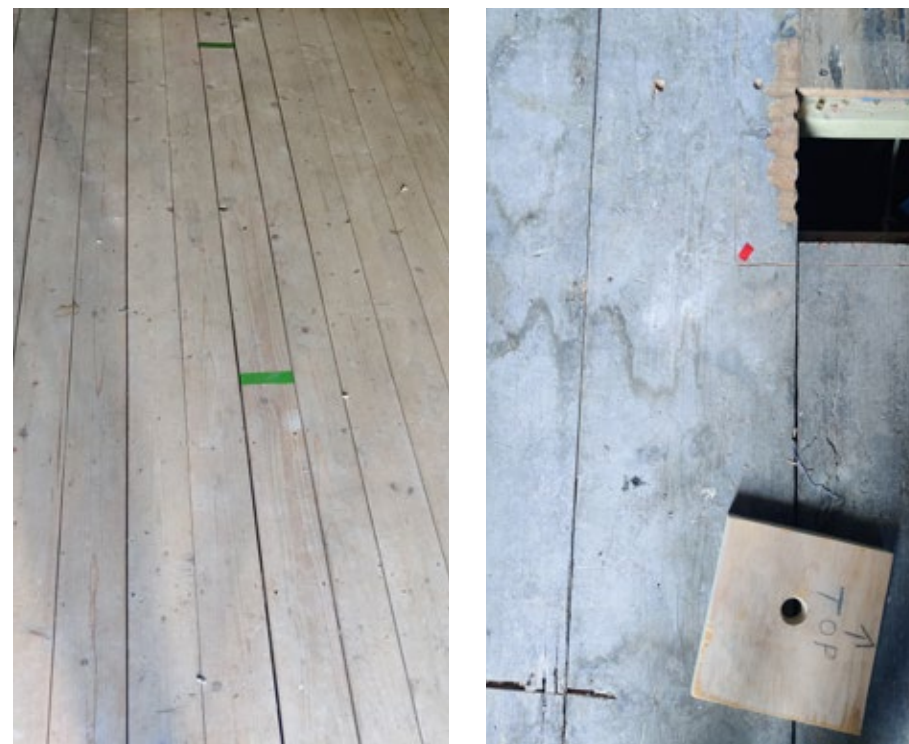
FIGURE 28. 794-F-04 Existing Floor Finish To Be Retained
