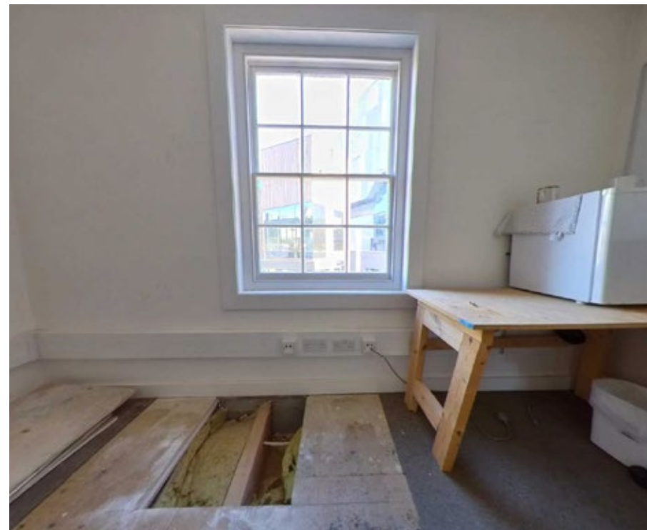
FIGURE 26. 792-F-06 No Evidence Of Floorboards
