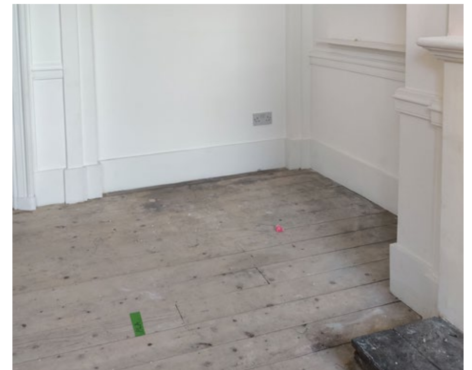
FIGURE 29. 794-F-05 Existing Floor Finish To Be Retained
