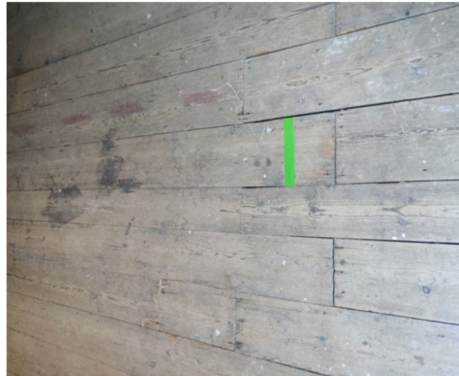
FIGURE 27. 794-F-03 Existing Floor Finish To Be Retained
