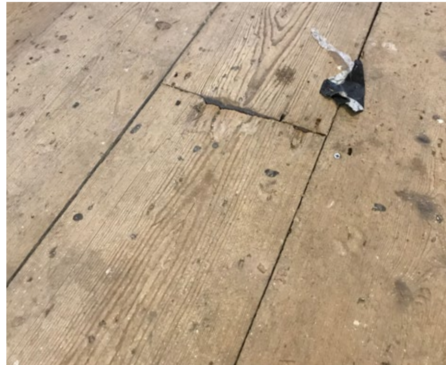
FIGURE 21. 794-G-01 Existing Floorboards in good condition
