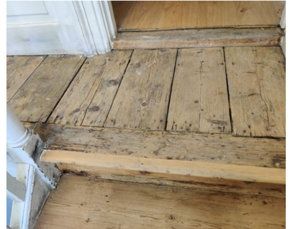
FIGURE 36. 794-S-01 Existing Floor Finish To Be Retained
