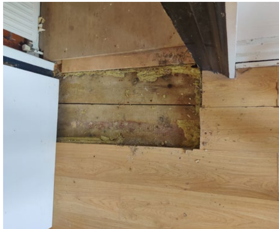
FIGURE 37. 794-S-04 Existing Floor Finish To Be Retained
