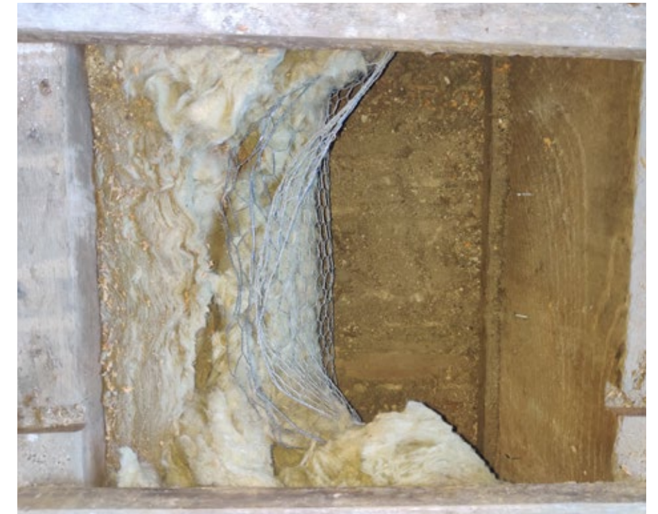
FIGURE 11. Lathe And Plaster Visible Through Historic Floor Boards On The First Floor Room Above
