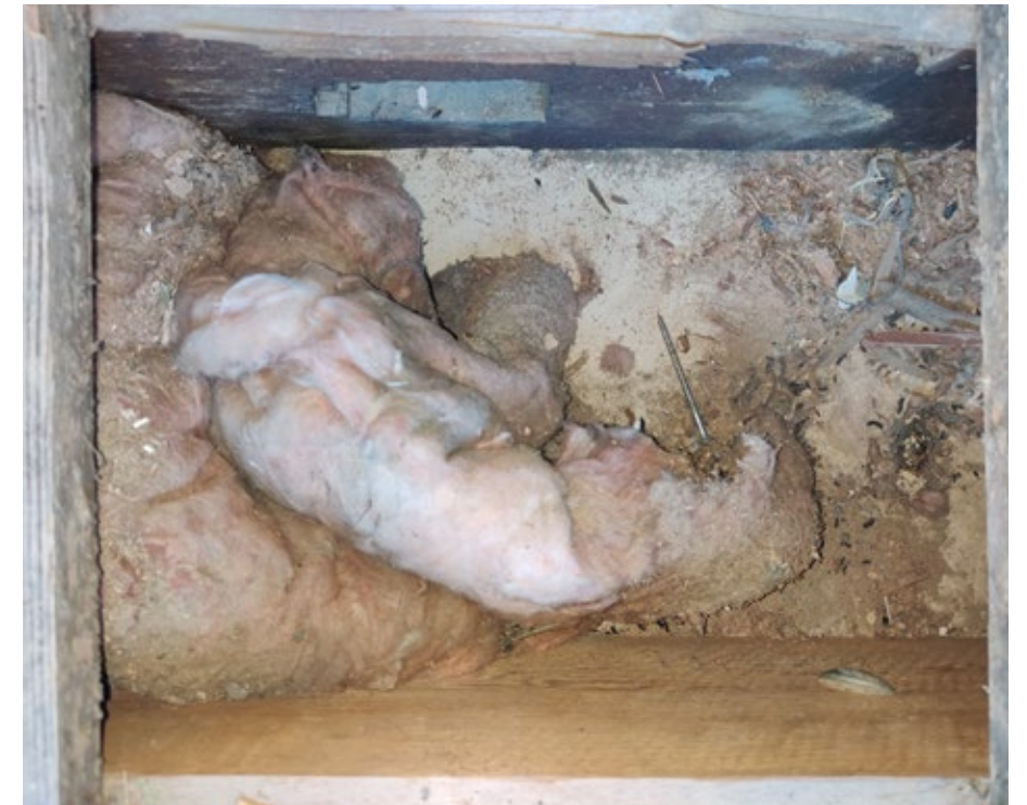
FIGURE 17. 794-G-05 Plasterboard Visible Through The First Floor Room Above
