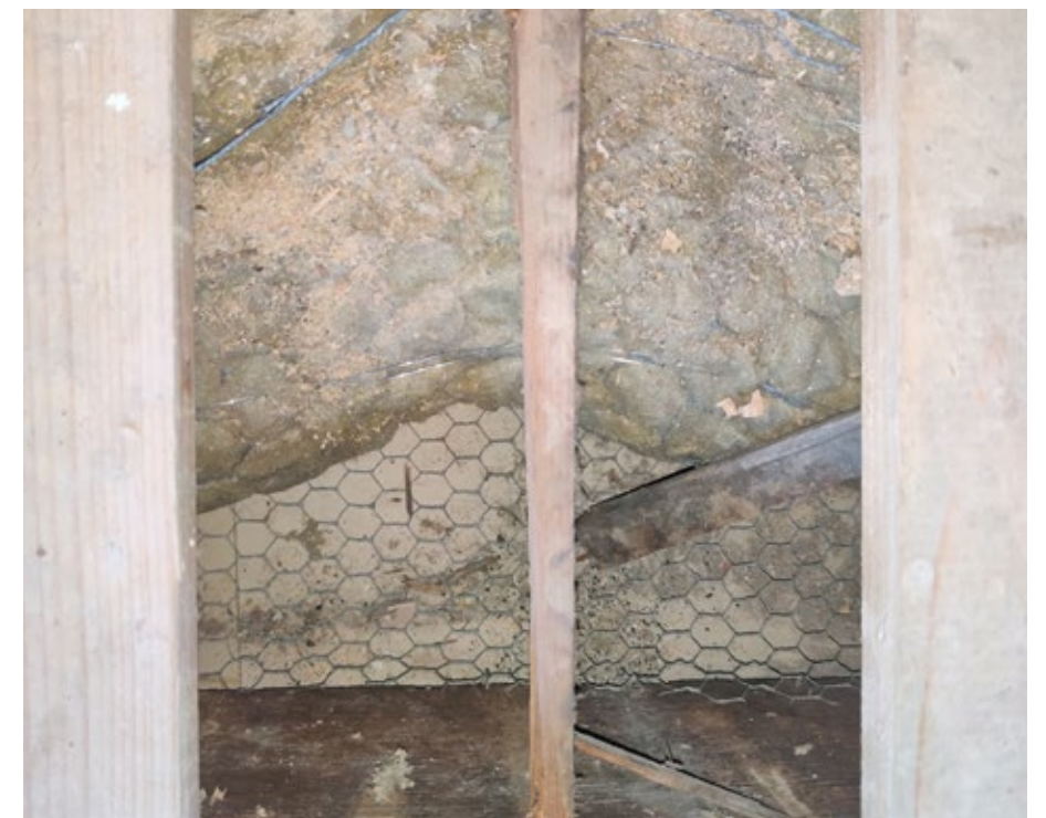
FIGURE 4. Existing Floor Boards Lifted
