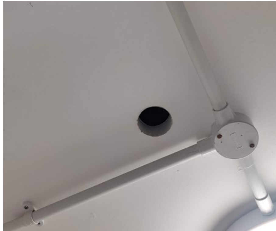
FIGURE 1. 50MM Core Hole
