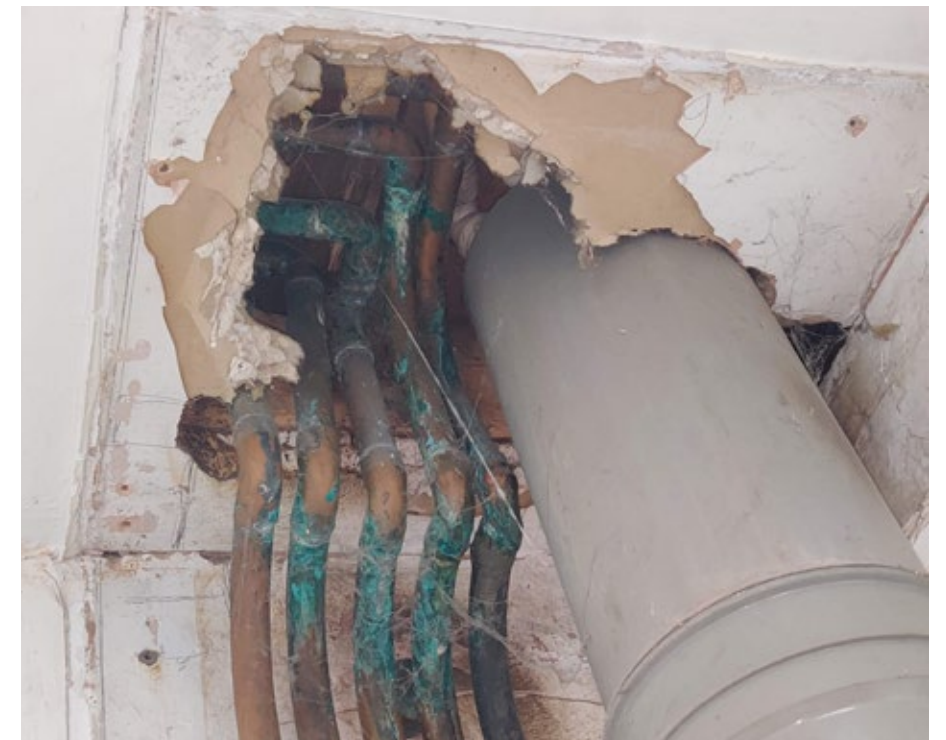
FIGURE 18. 792-B-05 Plasterboard Evidently Visible Through Existing Services Opening
