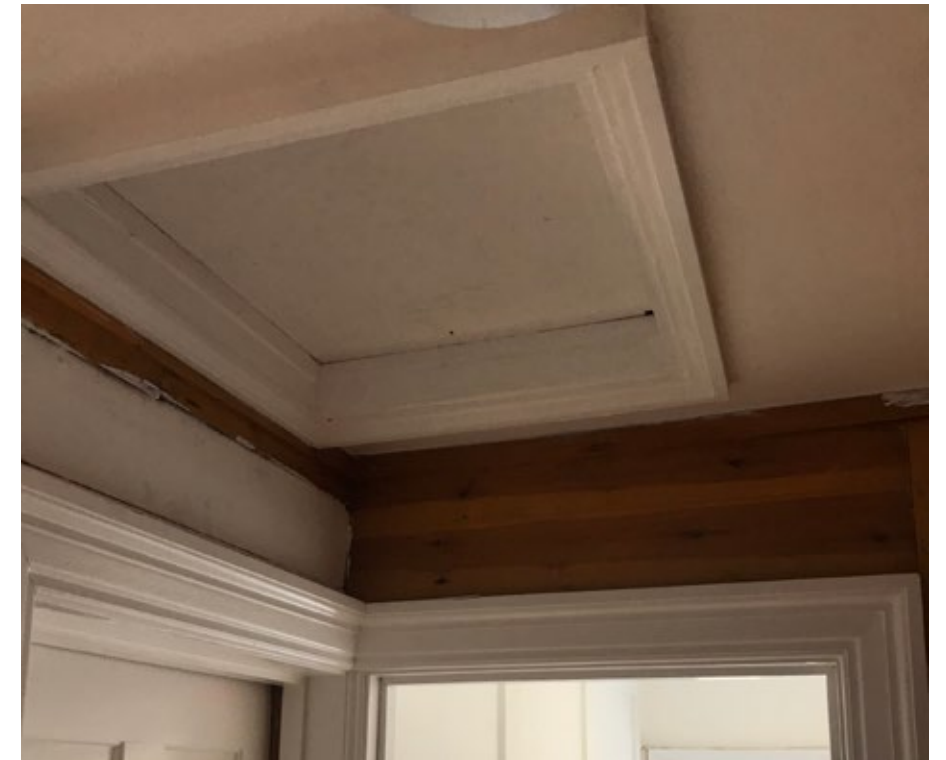
FIGURE 2. Existing Loft Hatch
