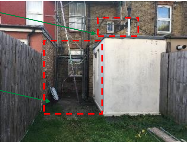
Photo 8: Typical existing modular pod and location of proposed kitchen extension.
