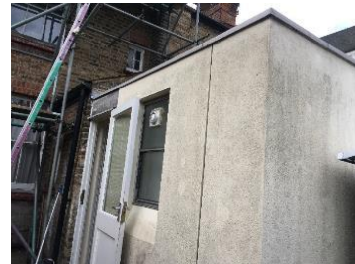
Photo 6: Side elevation of a pod
