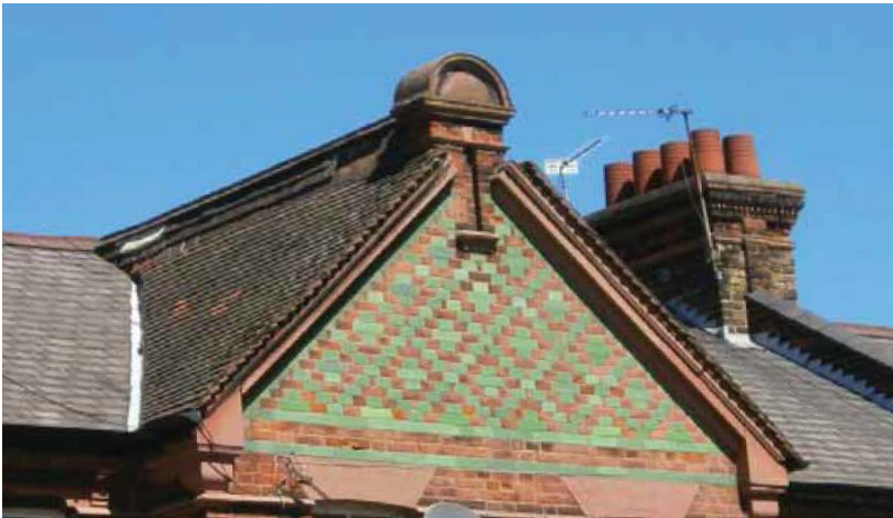
Photo 4: An example of a roof detail and the green bricks
