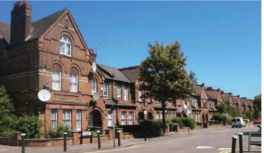
Photo 1: Gladstone Avenue Facade
