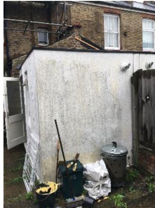
Photo 5: Typical existing modular pod.
