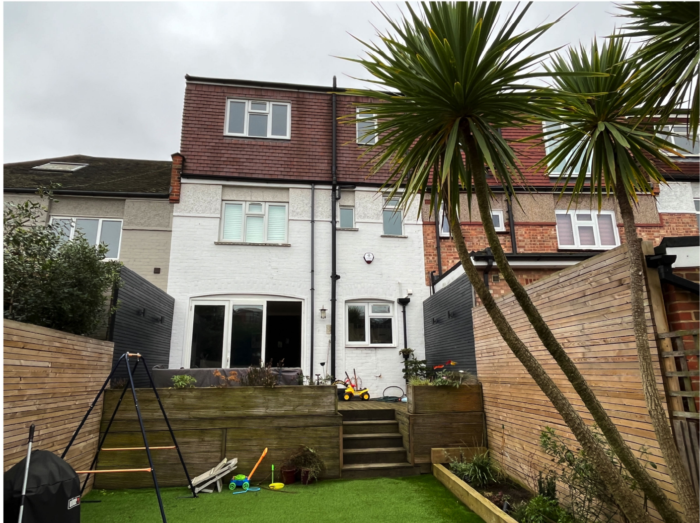
View of Rear Elevation from the Garden
