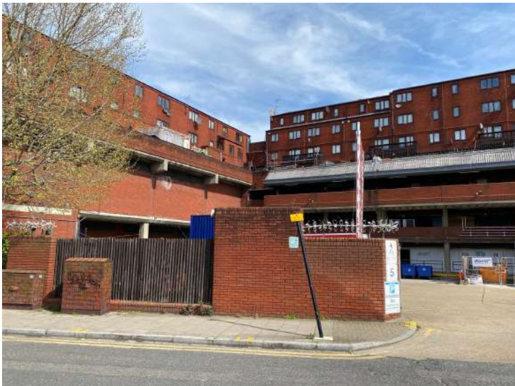
External view of site for new generator enclosure from Mayes Road
