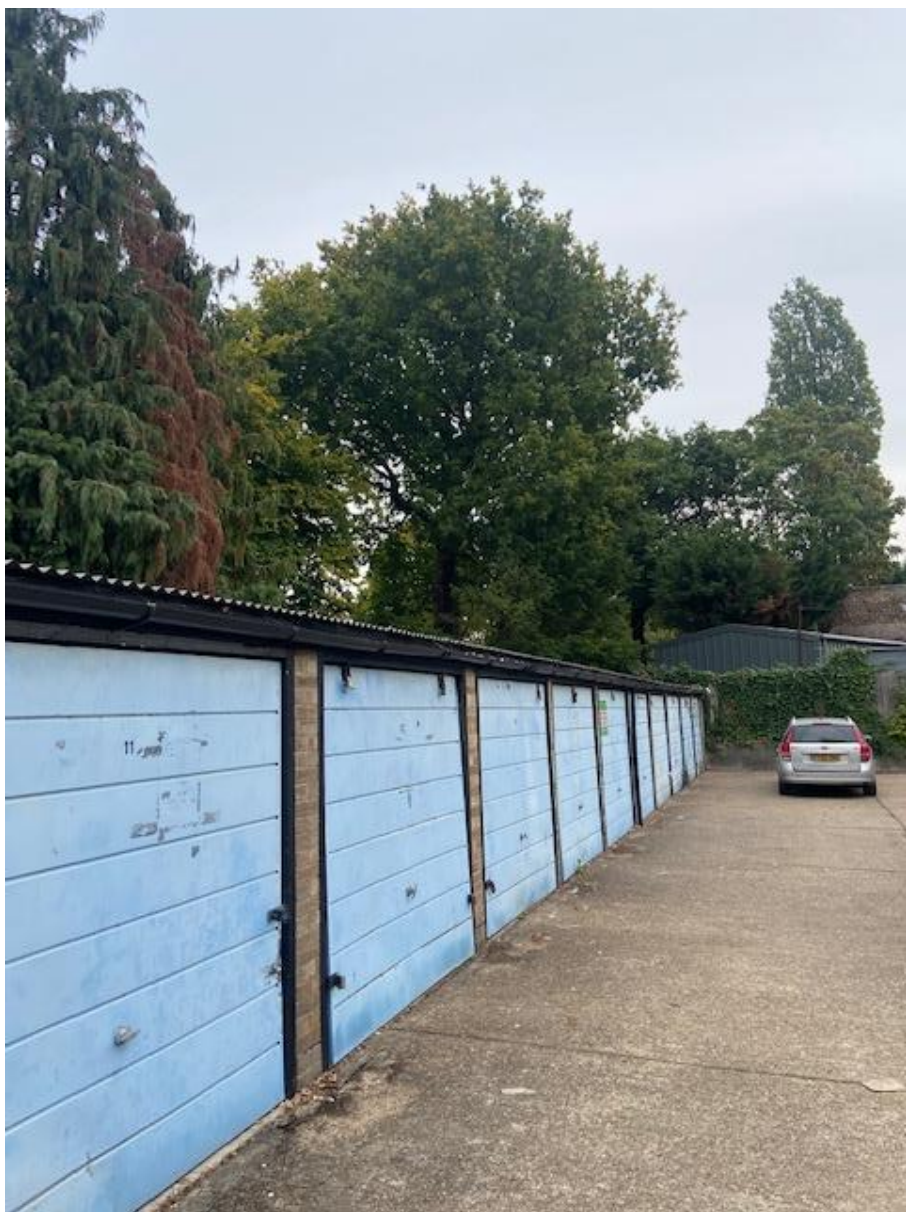
Northern block of garages
